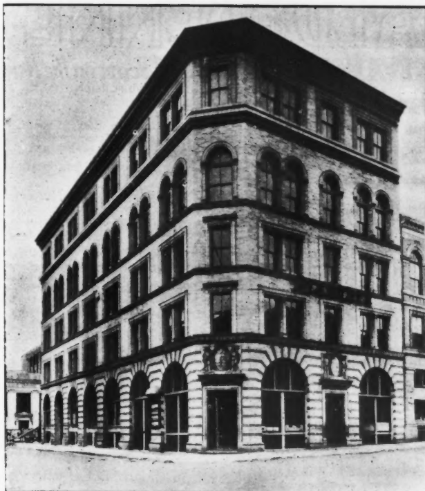
New plant of "New Bedford Standard" and the "Mercury."
