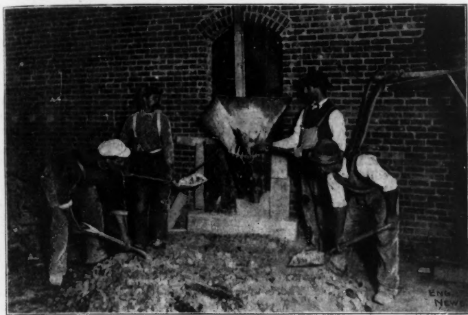
Fig. 1.—Shoveling the Material into the Hopper.
