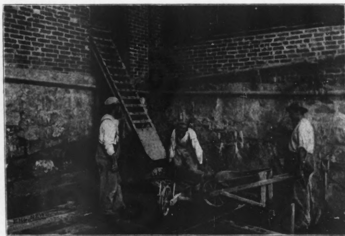
Fig. 2.—Controlling the Water and Wheeling Away the Concrete.
