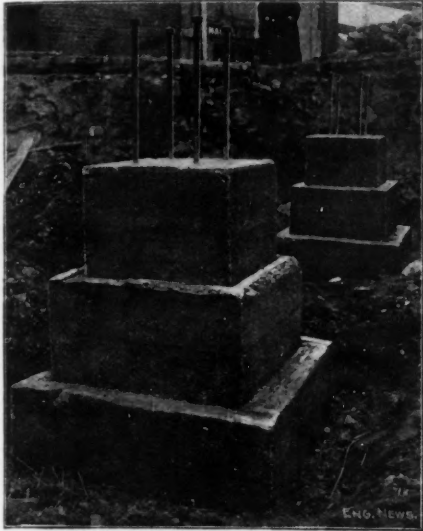
Fig. 2.—Column Foundation for Boston Elevated Railway, Uncovered, to Show Masonry.
