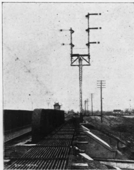
Fig. 5.—Steel Signal Post; C. M. & St. P. Ry. W. H. Elliott, Designer.
