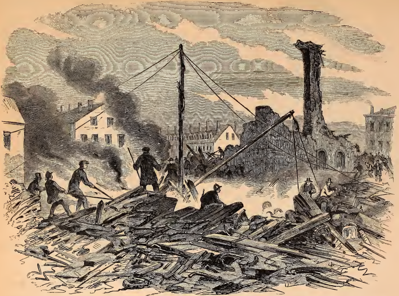
VIEW OF THE RUINS OF THE FREMONT MILLS, AT LAWRENCE, MASS., WITH POWERFUL DERRICKS ERECTED FOR THE PURPOSE OF REMOVING THE LOGS AND TIMBER, IN ORDER TO REACH THE BODIES OF THE VICTIMS BENEATH THE RUINS.—SEE PAGE 130.
