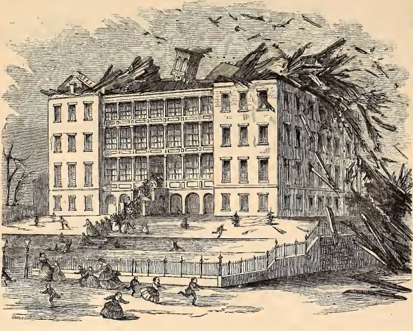
UNROOFING OF THE CATHOLIC ORPHAN ASYLUM, ON FIFTY-FIRST STREET AND FIFTH AVENUE—THE BUILDING SERIOUSLY DAMAGED—RESCUE OF THE CHILDREN.
