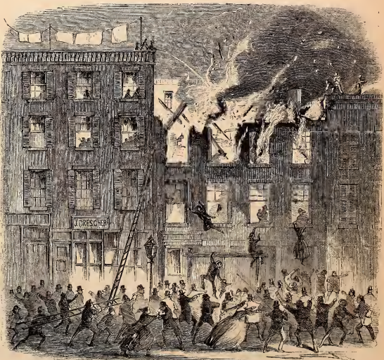
WRECKFUL FIRE AT NO. 205 BAYVIEW STREET, NEW YORK, ON TUESDAY MORNING, JANUARY 3RD—SIX LIVES LOST BY FIRE AND SUFFOCATION.—FROM A SKETCH BY OUR OWN ARTIST.
