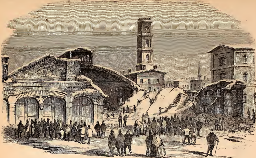
VIEW OF THE UNION RAILROAD DEPOT, TROY, N. Y., AFTER THE FALLING OF THE ROOF AND WALLS ON THE NIGHT OF THE 30TH OF DECEMBER, 1859.—FROM A PHOTOGRAPH BY CLARKE & HOLMES, TROY.
