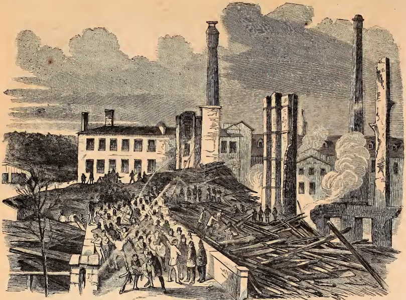
FIERCELY CALAMITOUS—FALLING OF THE PEMBERTON MILLS AT LAWRENCE, MASS.—VIEW OF THE RUINS OF THE PEMBERTON MILLS, LOOKING TOWARDS THE MERRIMAC—FROM A SKETCH TAKEN ON THE SPOT BY OUR OWN ARTIST.
