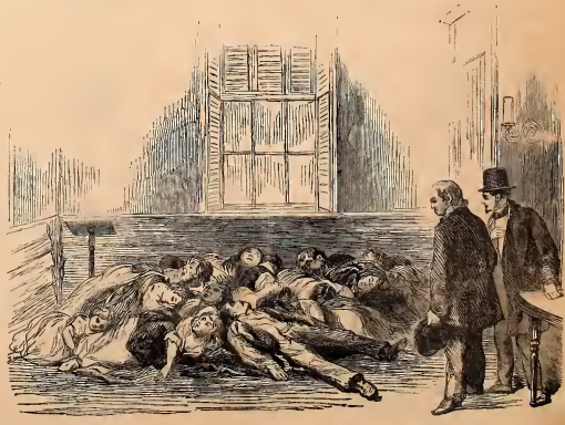
VIEW OF THE ROOM ADJOINING THE LABOR HALL, IN THE CITY HALL, CONTAINING THE DEAD BODIES OF DECEASED SUFFERERS SACRIFICED BY THE FALLING OF THE PENNSYLVANIA MILLS.
