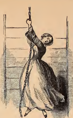
WONDERFUL ESCAPE OF MISS OLIVIA BRIDGES—HEARING THE CRASHING OF THE BUILDING, SHE RAN TO THE ROPEWAY, DESCENDED BY THE CHAIN, FIVE STORIES, AND ESCAPED.—SEE PAGE 122.
