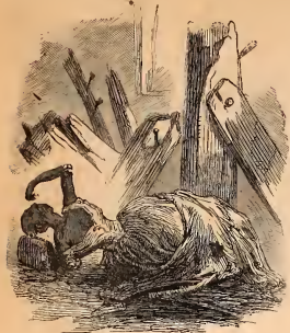
APPEARANCE OF ONE OF THE BODIES IMMEDIATELY AFTER IT WAS TAKEN FROM THE BOOMS OF THE FAMBERTON MILLS.
