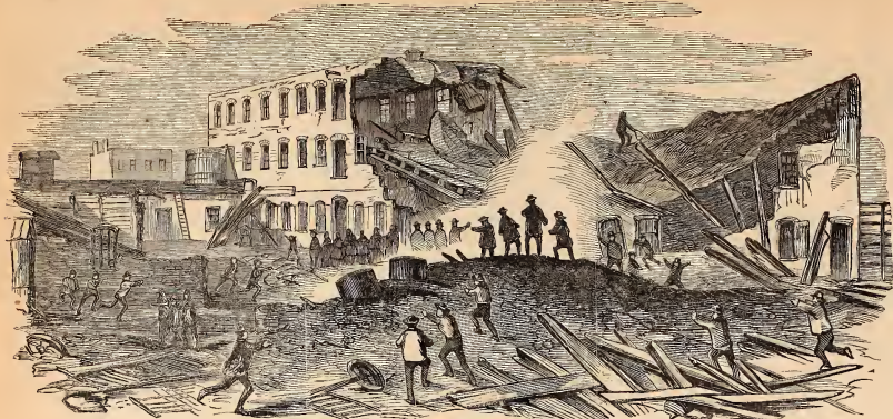
TERRIBLE EXPLOSION AT AMES & MOULTON'S HAT MANUFACTORY, COR. OF SANFORD STREET AND MYRTLE AV., EAST BROOKLYN, ON FRIDAY, FEB. 3RD.—TWENTY OR THIRTY PERSONS KILLED AND WOUNDED.
