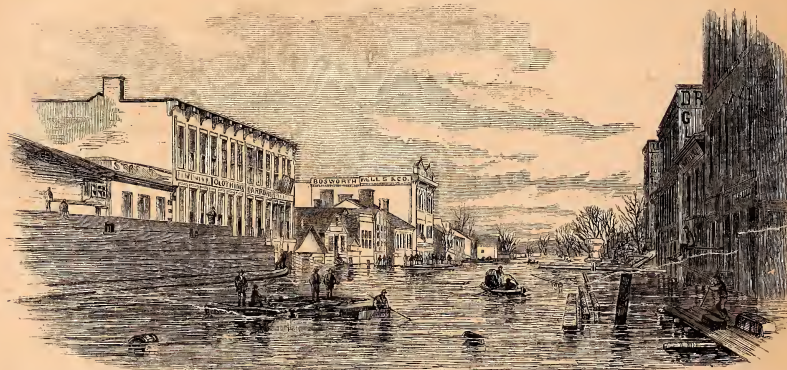
VIEW IN FRONT STREET, MARIETTA, OHIO, ON THE MORNING OF THE FLOOD.—PHOTOGRAPHED BY E. S. HOLLISTER.
