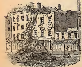
BONDED WAREHOUSE IN WEST STREET ENTIRELY UNROOFED.
