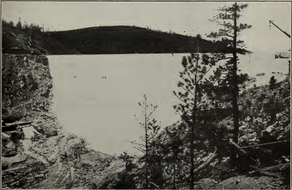
FIG. 2.—LOWER VIEW OF THE GIGANTIC CONCRETE DAM WHICH HOLDS BACK 525 MILLION CUBIC FEET OF WATER IN BOULDER CANYON, COL.
