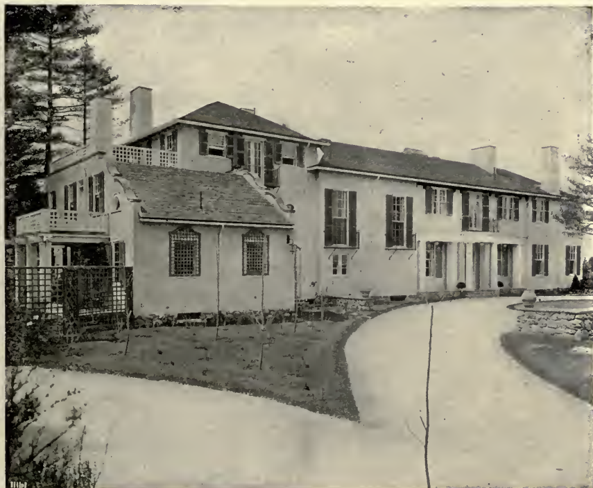
DOORWAY AND APPROACH
