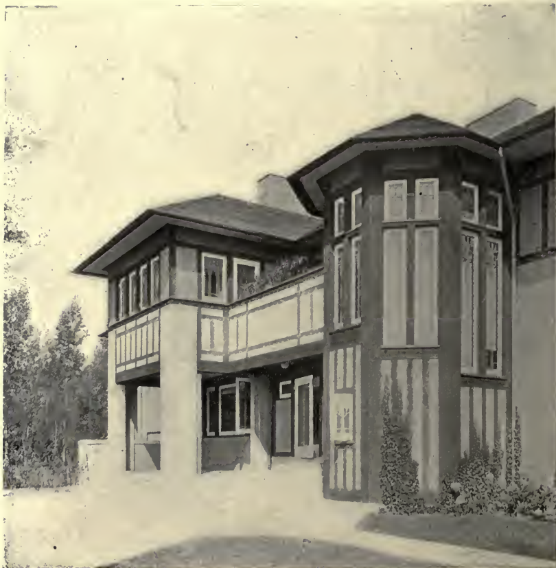
A SIMPLE TREATMENT OF BRICK AND PLASTER
