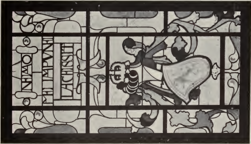
LEADED WINDOW, WITH THE PATTERN ETCHED HERE AND THERE, AS ON THE CROWN AND SHIELD
