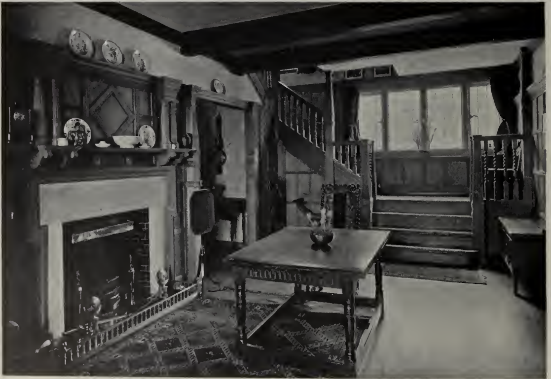
THE HALL, TOYS HILL, KENT. THE PANELLING AND FLOOR ARE OF WAINSCOT OAK, AND THE STAIRS WERE BUILT UP WITH OLD BALUSTERS. THE MATERIALS USED IN THE BUILDING OF THE HOUSE WERE LYMPFIELD COURSED RAG-STONE AND HOWLEY PARK STONE, THE FIRST HAVING A RICH YELLOW TONE, THE OTHER A STRONG GREY
