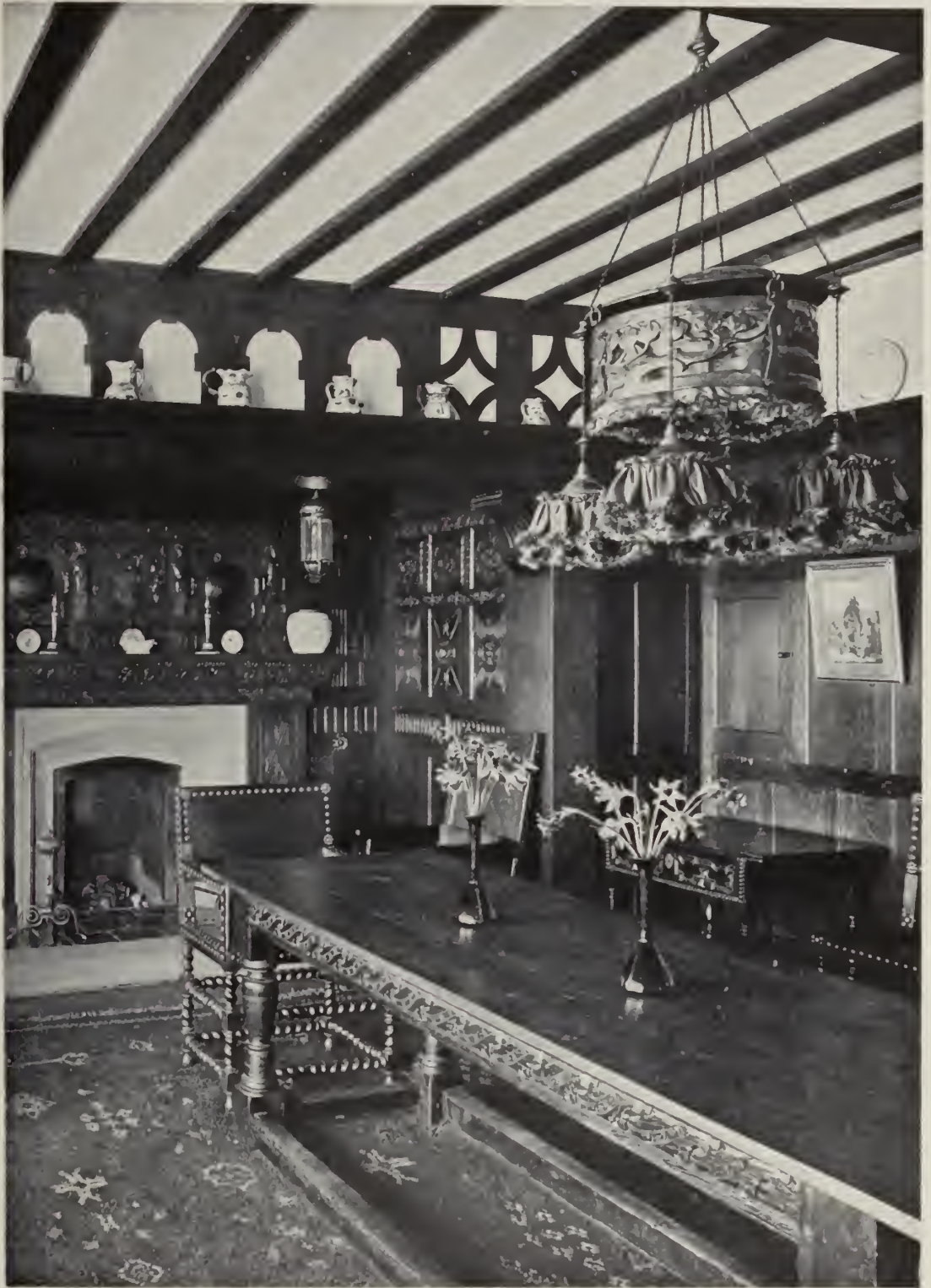
VIEW OF THE DINING-ROOM IN A HOUSE BUILT AT BARNT GREEN, WORCESTERSHIRE, FOR FRANK RABONE, ESQ. THE PANELLING AND THE CARVED-WORK ARE IN OAK; OAK AND PLASTER HAVE BEEN USED FOR THE FRIEZE; THE ELECTRIC FITTINGS, MADE BY THE BROMSGROVE GUILD, ARE OF COPPER; AND THE FIRE PLACE IS IN RED BROMSGROVE STONE. THE TABLES AND THE CHAIRS ARE OLD
