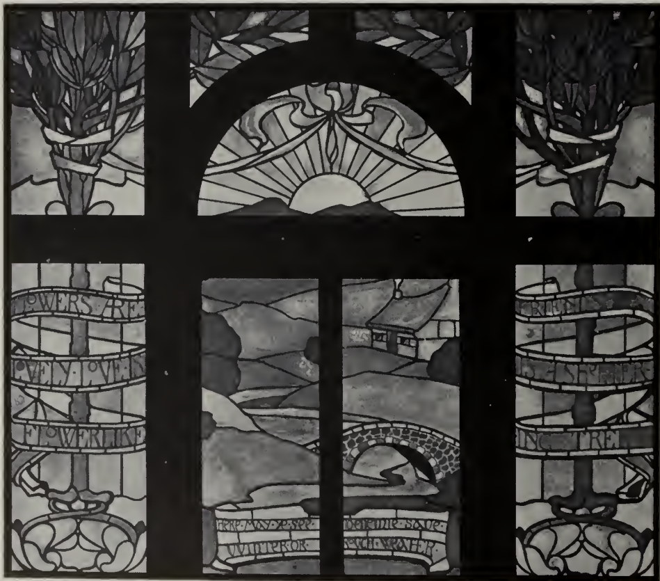
LEADED WINDOW WITH OLIVE AND DARK GREEN TREES. THE SETTING SUN IS REPRESENTED BY A PIECE OF ROUGH-CAST PLATE GLASS WITH A BEVELLED EDGE. THE RAYS ARE CARRIED OUT BY MEANS OF ALTERNATING STRIPS OF WHITE FLUTED GLASS, AND OF FLAT GLASS STAINED YELLOW
