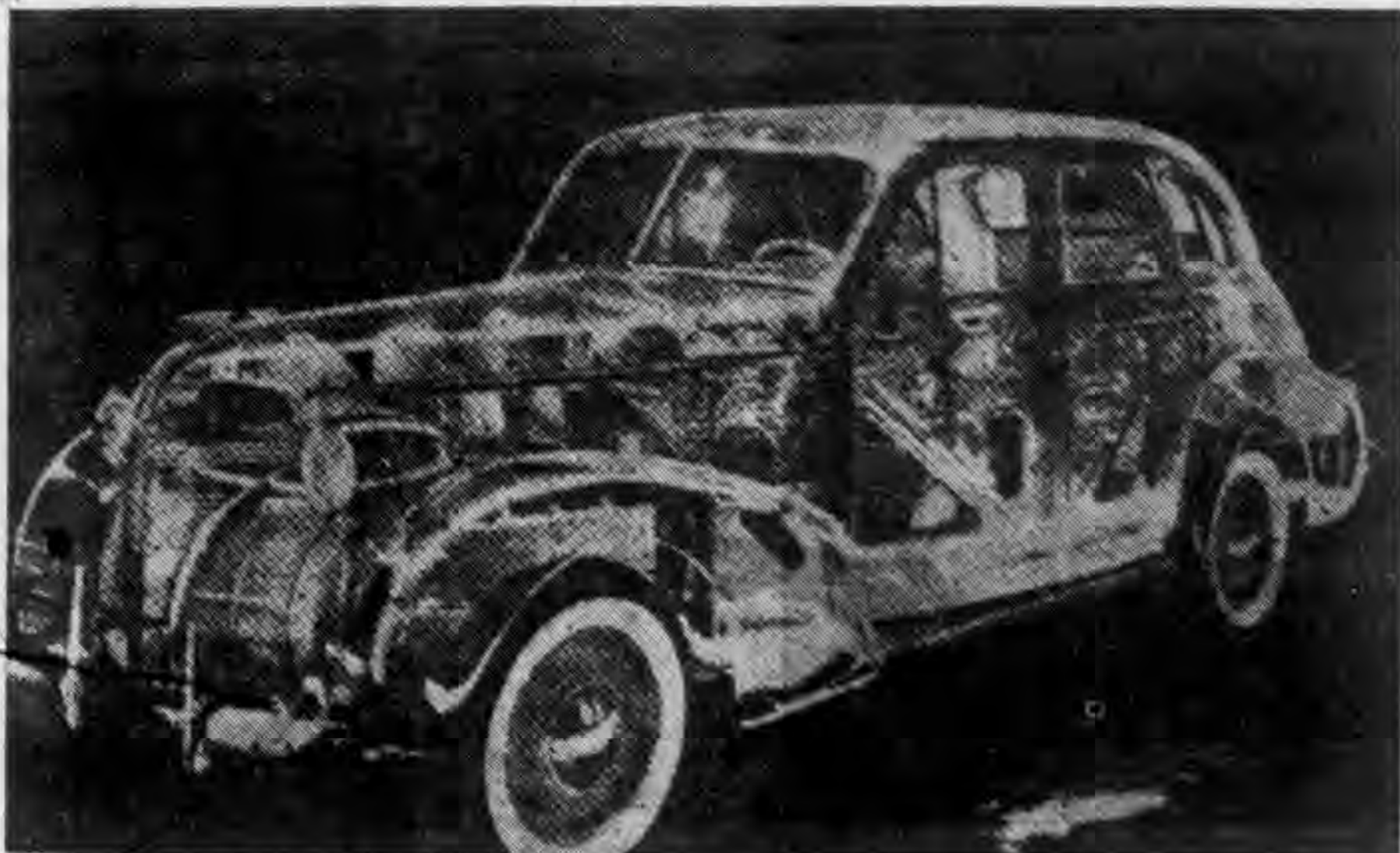
○然原目一，造構之圖機部內，車汽之成製膠樹用2
