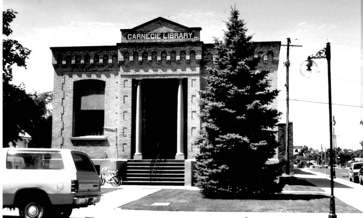
Ritzville Historic District, Ritzville, Adams Co., WA Photo #2.
