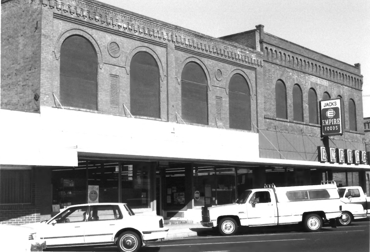
Ritzville Historic District, Ritzville, Adams Co., WA Photo # 6
