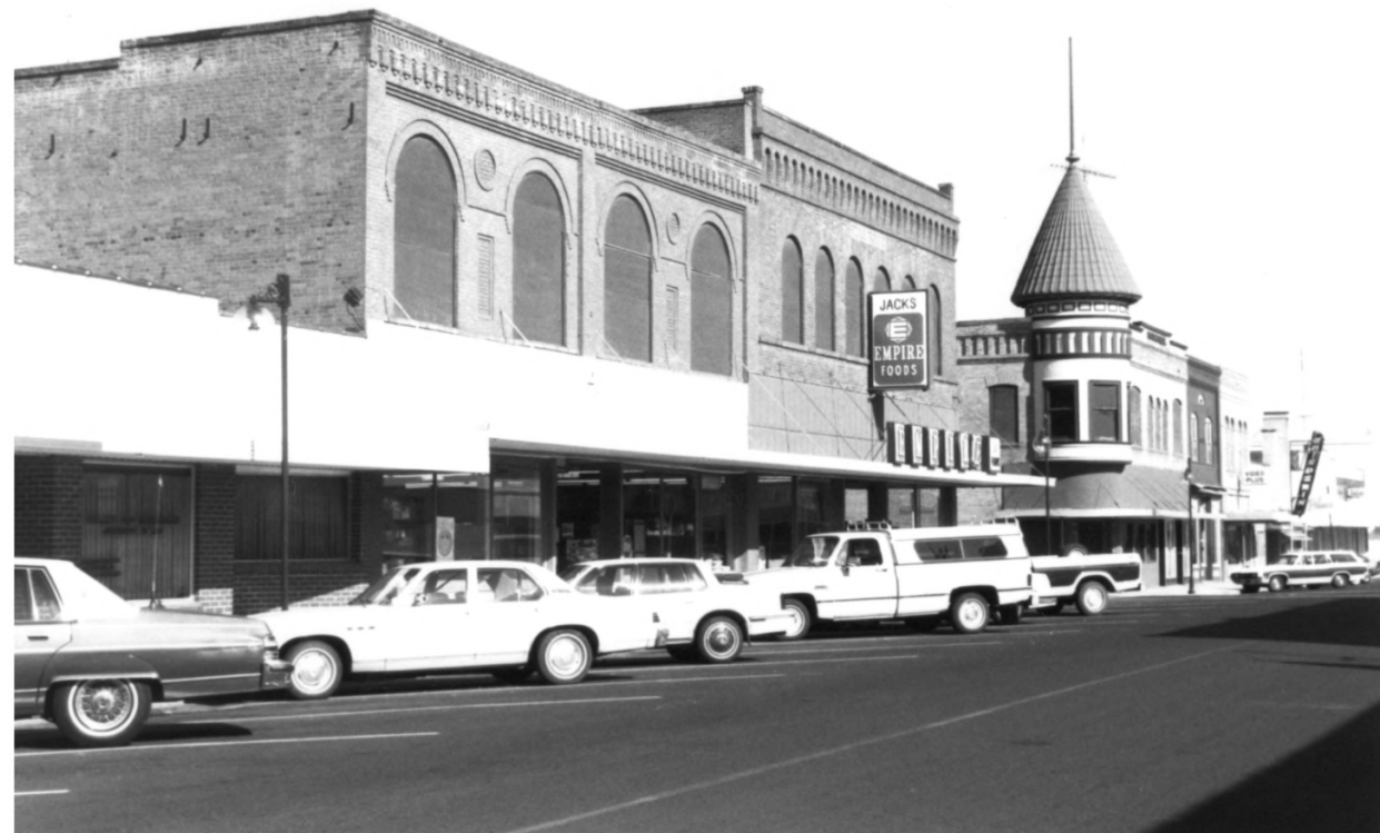
Ritzville Historic District, Ritzville, Adams Co., WA Photo #5
