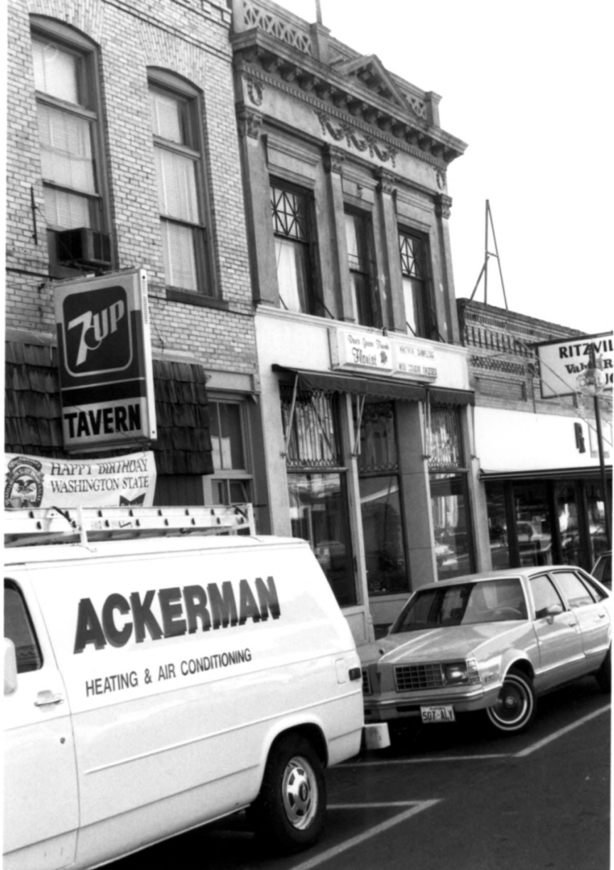
Ritzville Historic District, Ritzville, Adams Co, WA Photo #20
