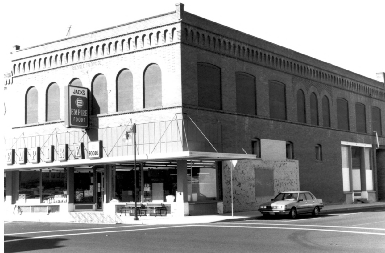
Ritzville Historic District, Ritzville, Adams Co., WA Photo # 7
