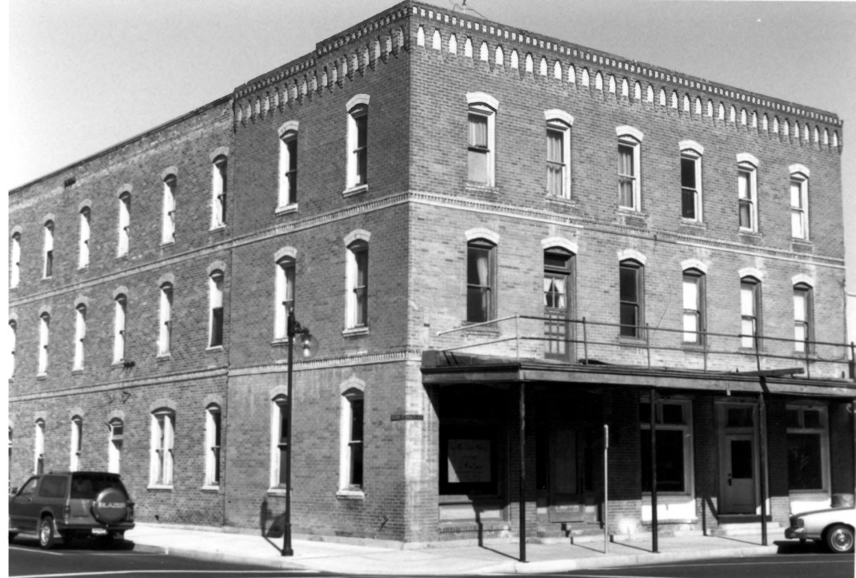
Ritzville Historic District, Ritzville, Adams Co., WA Photo #4
