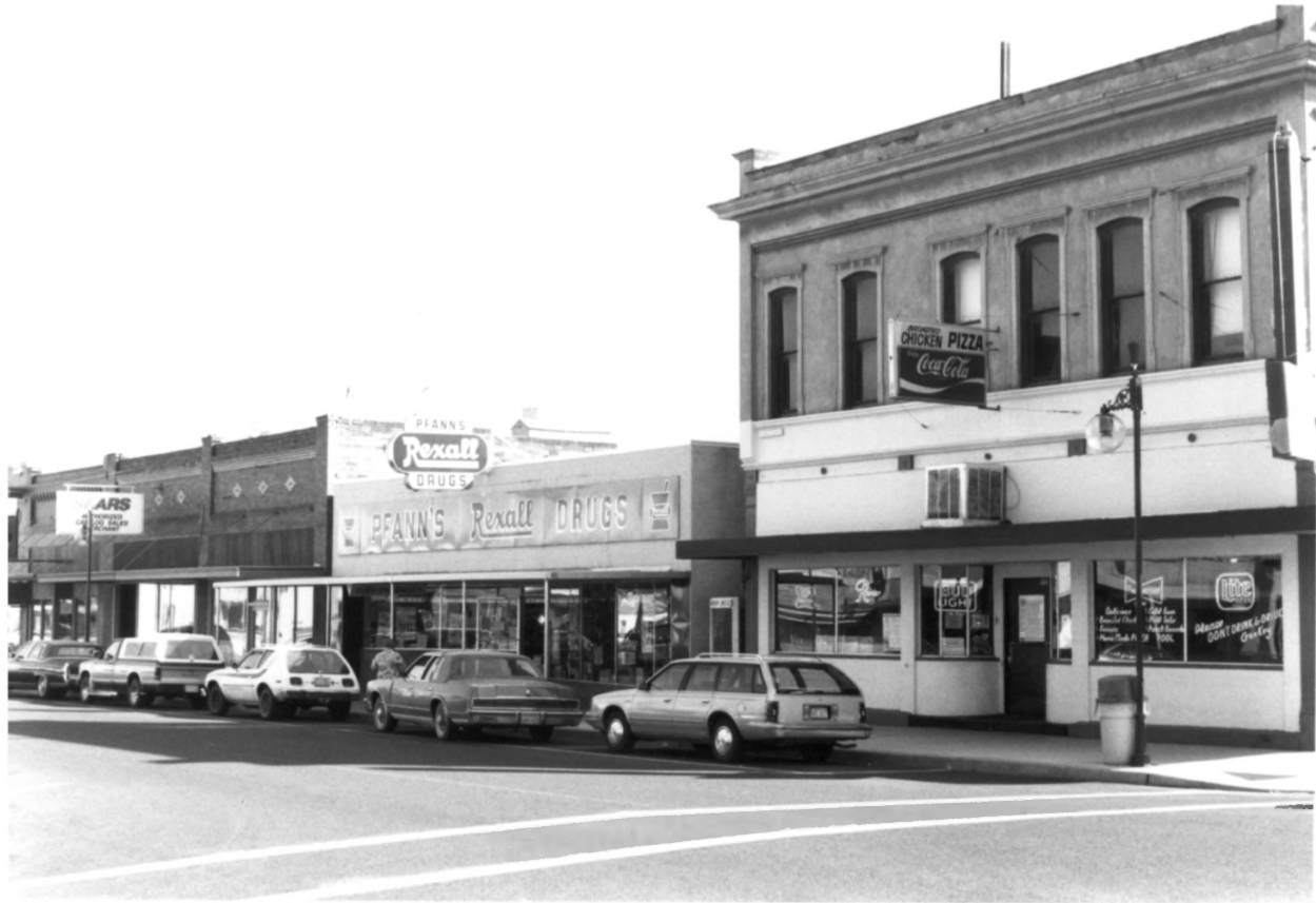
Ritzville Historic District, Ritzville, Adams Co., WA Photo # 16
