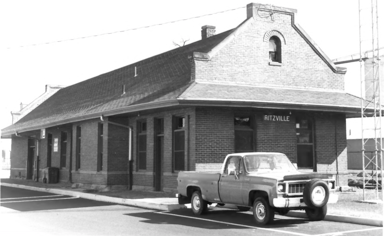
Ritzville Historic District, Ritzville, Adams. Co, WA Photo # 27
