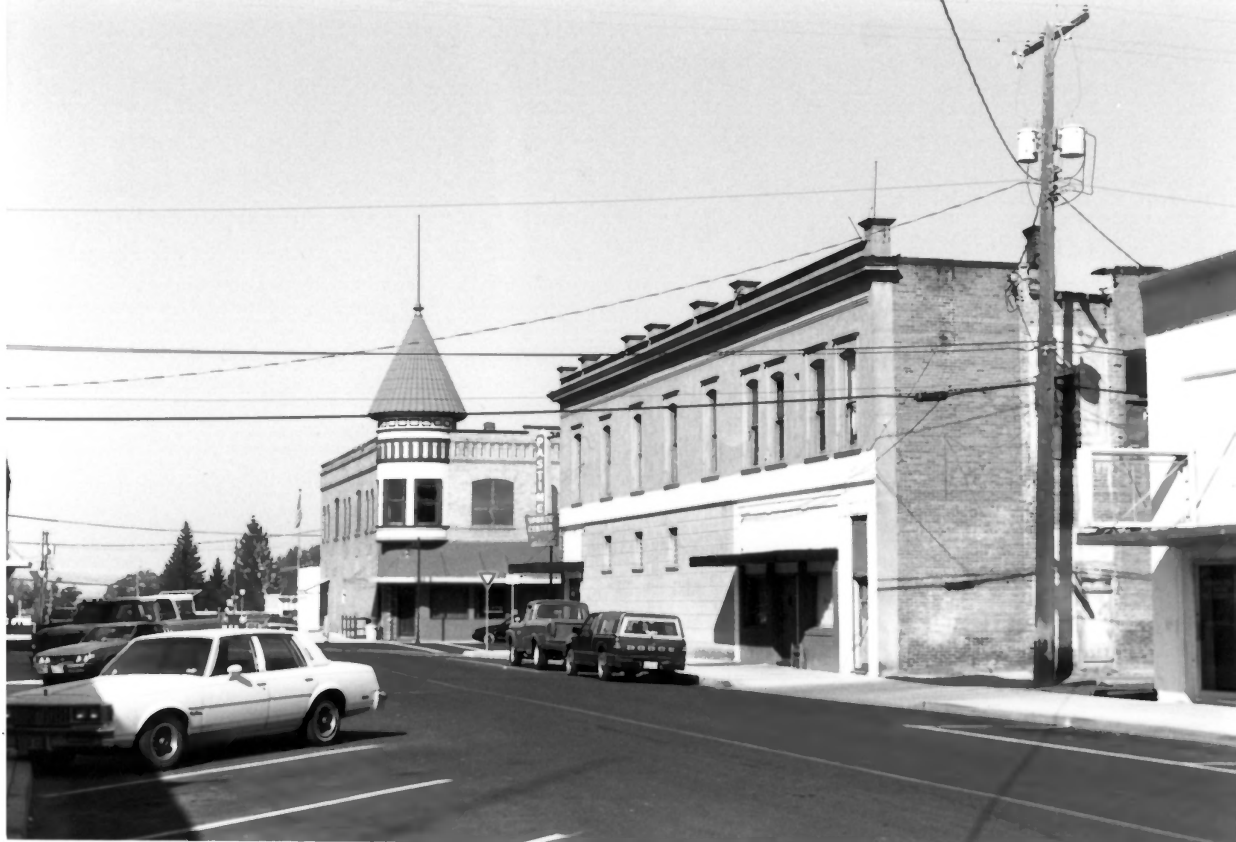
Ritzville Historic District, Ritzville, Adams Co., WA Photo # 18
