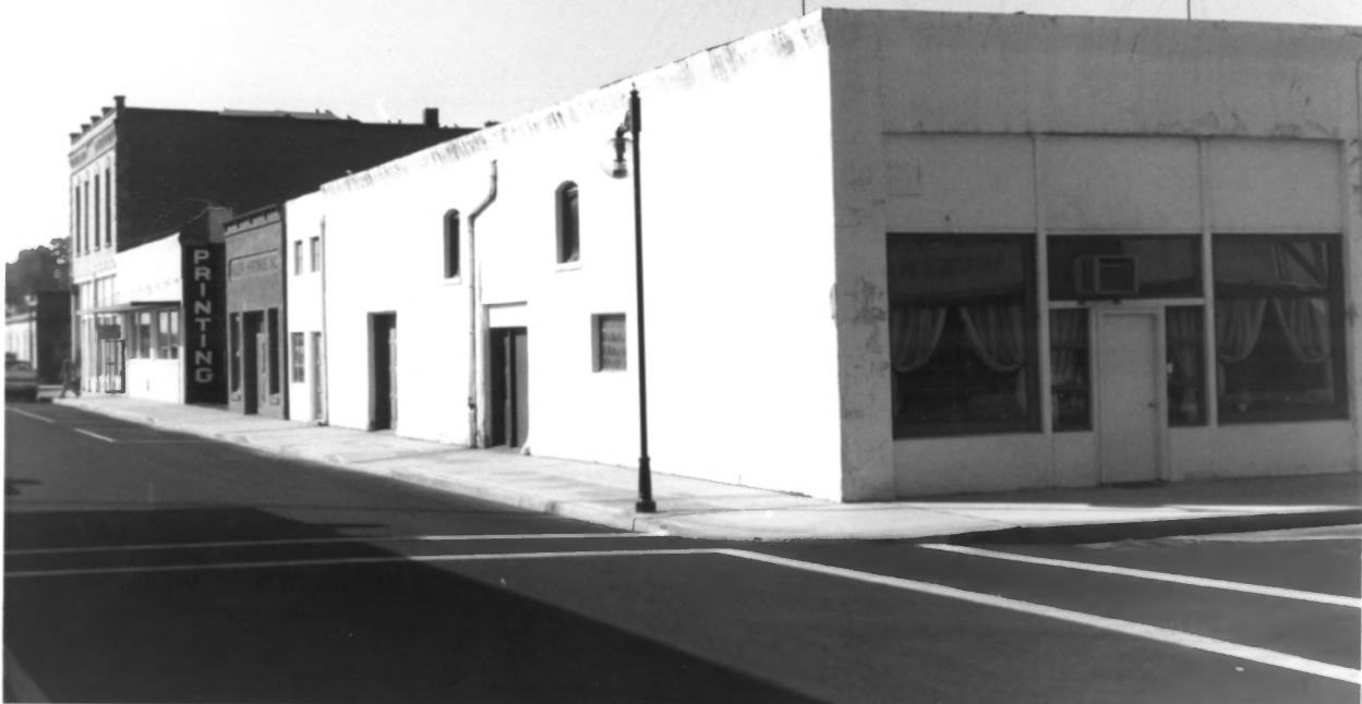
Ritzville Historic District, Ritzville, Adams Co., WA Photo # 26
