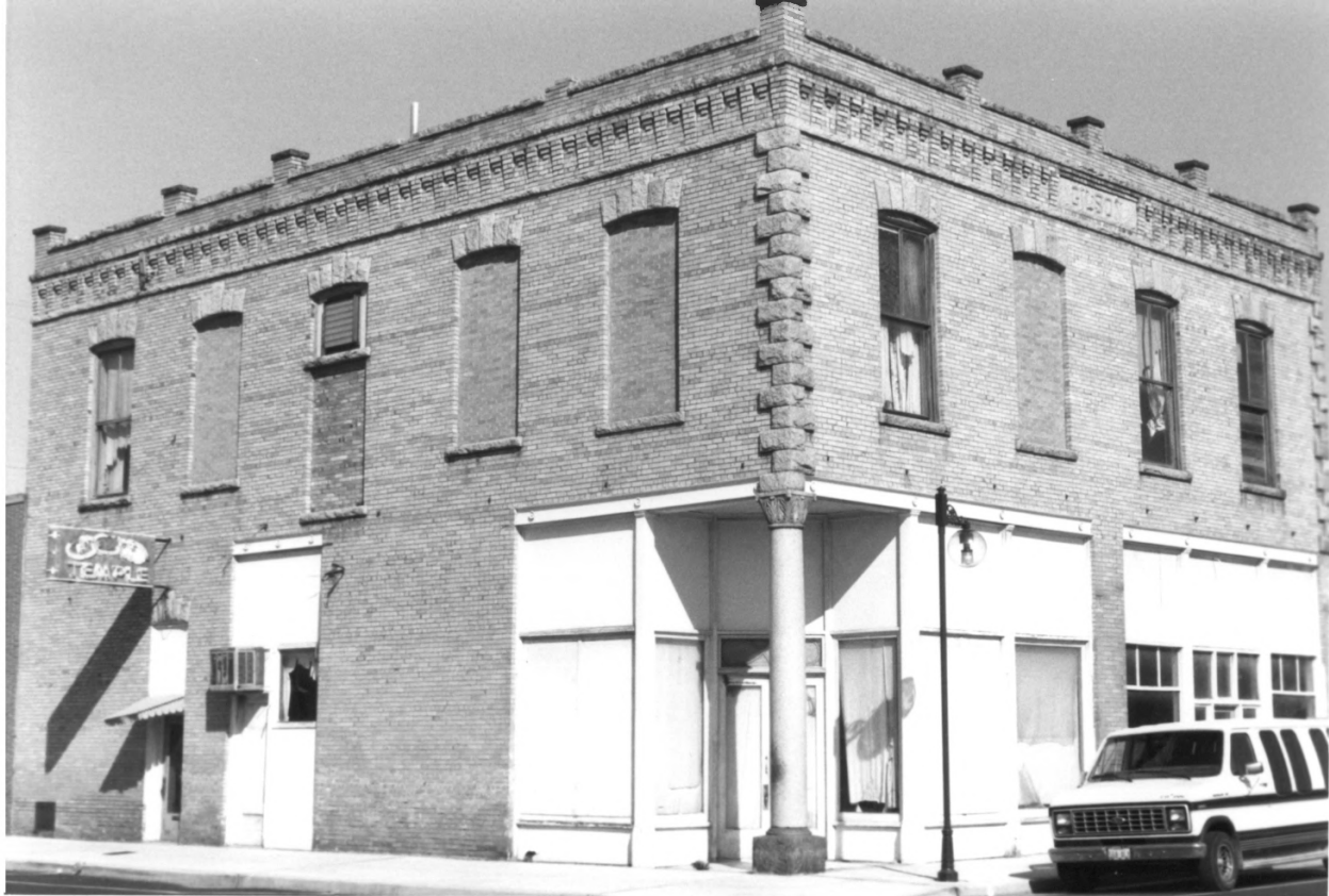
Ritzeville Historic District, Ritzeville, Adams Co., WA Photo #24
