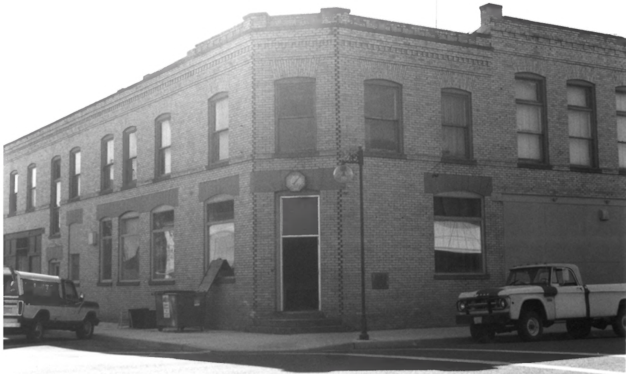
Ritzville Historic District, Ritzville, Adams Co, WA Photo #19
