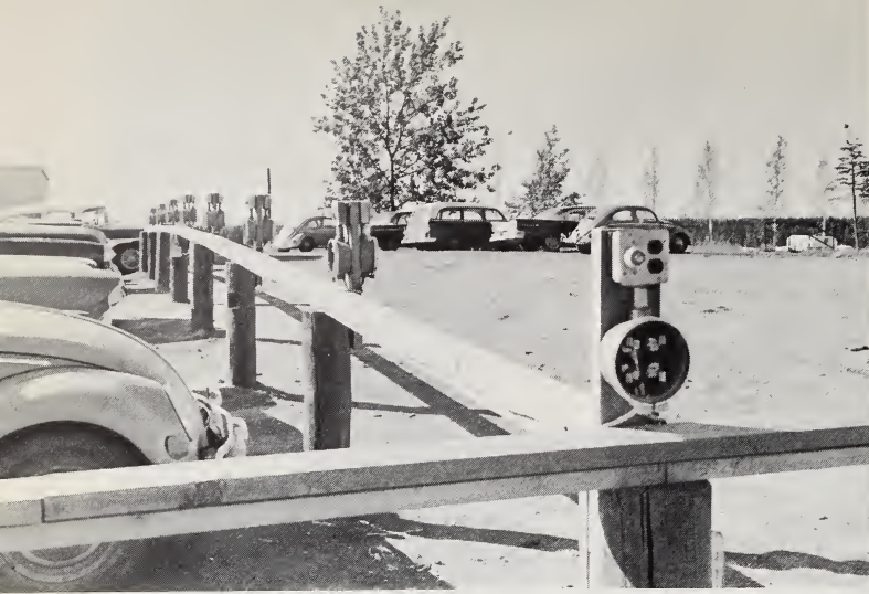
These outlets for headbolt heaters at the University of Alaska are served by Golden Valley, of Fairbanks.
