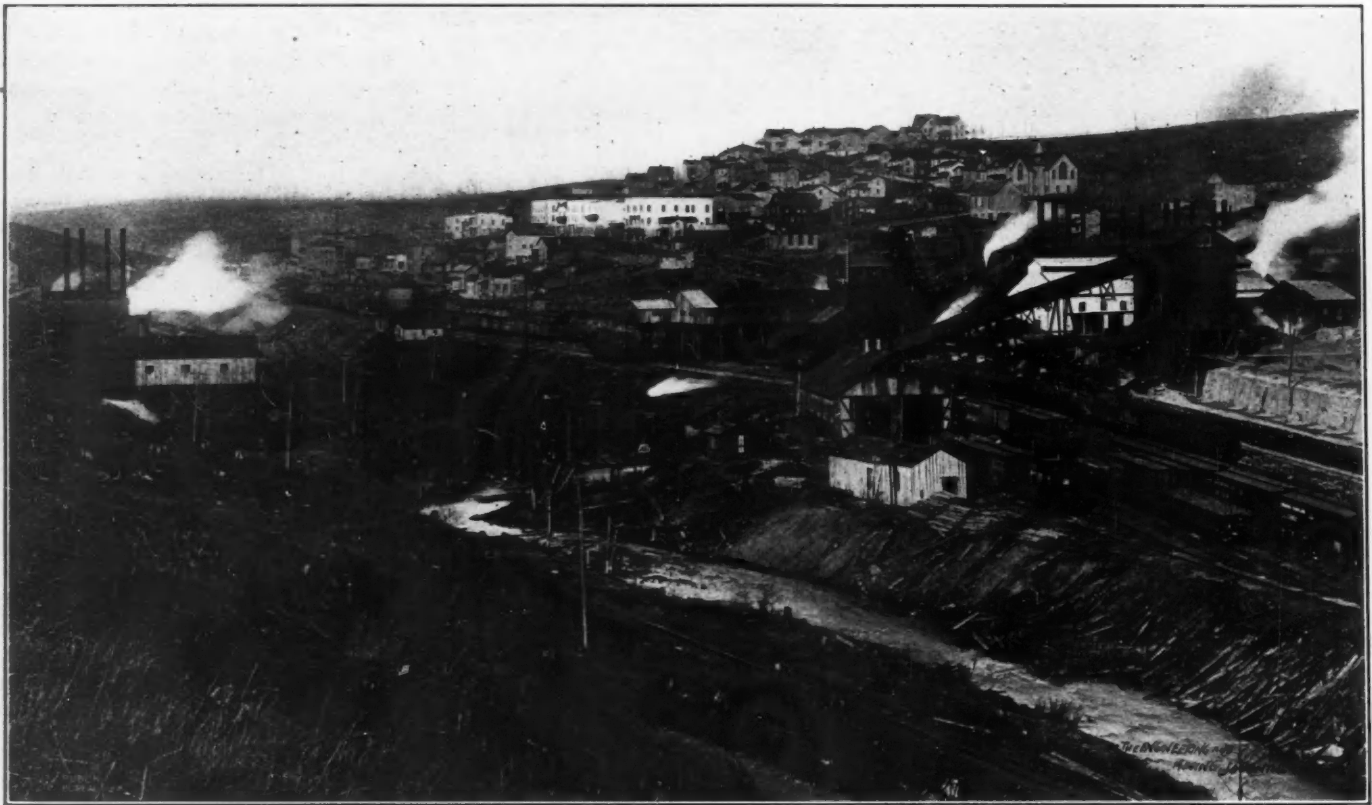
GENERAL VIEW OF THE THOMAS POWER PLANT AND TIPPLES BELONGING TO THE DAVIS COAL AND COKE COMPANY
