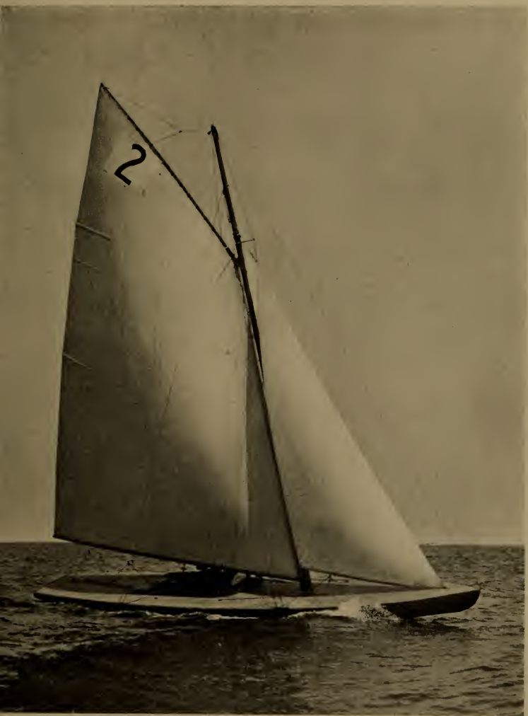
Narrow, scow formed Sonder boat with long, straight side. She was second choice for the American team of 1906. A good example of the high, narrow rig
