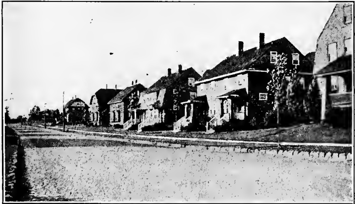
Well Planned Street of Double Family Houses, Hopedale, Mass., Renting from $16.00 to $18.00
