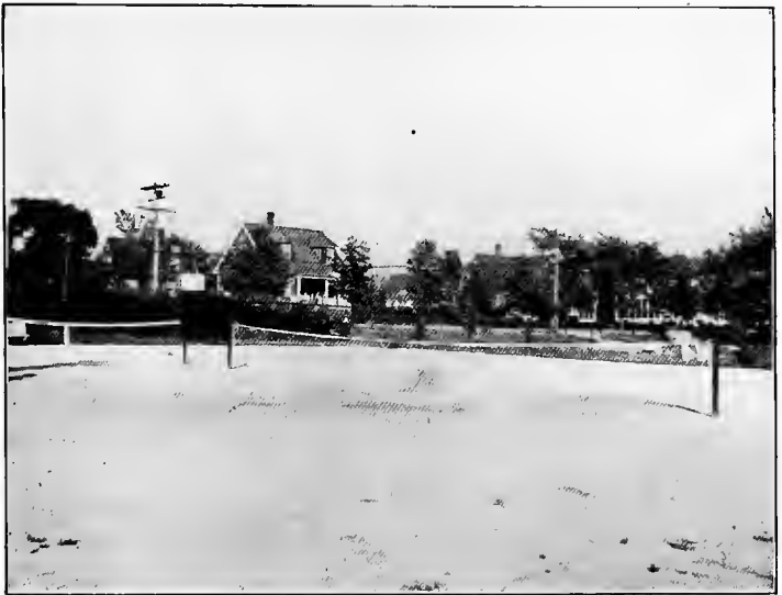
Town Tennis Courts, Francis William Park, East Walpole
