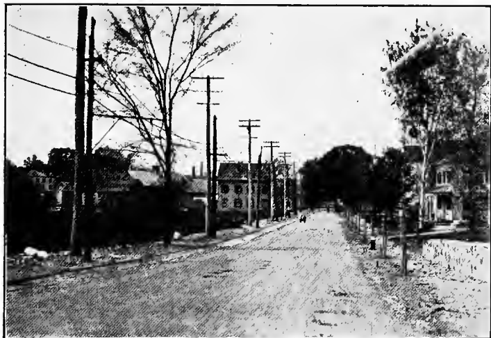
East Street, Walpole, Mass., Showing Ugly Telegraph Poles
