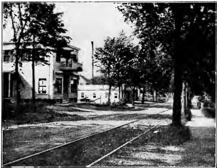
Washington Street, East Walpole. Present Width 49 Feet. Example of the Crowding which Is Piling Up Bills for the Future. Foot Building Line.
