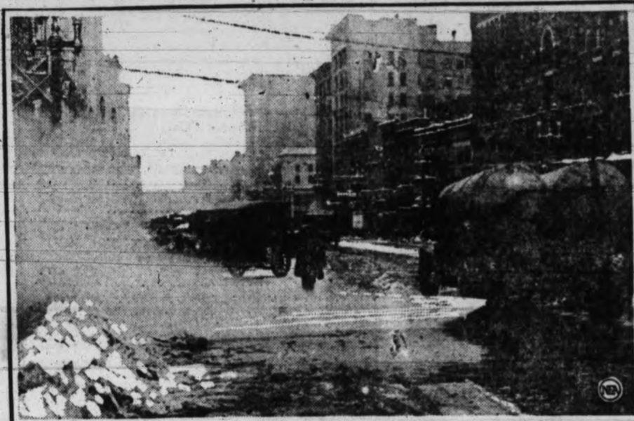
CONQUERING THE SNOW KING. —In Salt Lake City they use hot water to flush the streets when snow impedes progress. Heating the water doesn't cost the city a cent, either, since it's piped from natural springs at 110 degrees Fahrenheit. Photo shows a municipal sprinkler pulling the fire away from a lane of the wintery stuff.
