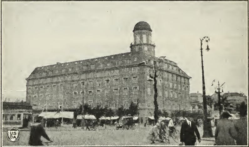
FIG. 22.—The building owned and occupied by the Danish Cooperative Bank, Copenhagen. The capital stock is owned by the various cooperative associations in the country.
