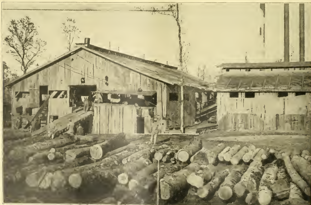
THIS WAS ERRECTED BY THE 20th ENGINEERS NEAR ST. DIZIER AND SURPRISED THE FRENCH WITH ITS LARGE DAILY PRODUCTION, AS IN FACT DID ALL THE OTHER MILLS
