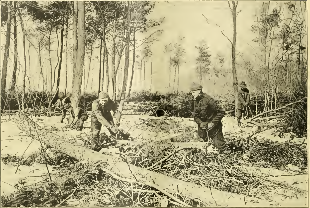
20th ENGINEERS SAWING FELLED TREES INTO LOGS IN A PINE FOREST, SOUTHERN FRANCE
