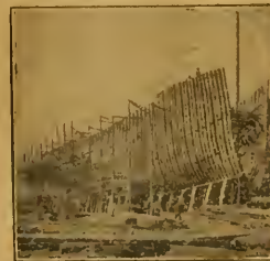
Faying surfaces of timbers brush-treated with Carbosota. (Courtesy Peninsula Ship Bldg. Co.)
