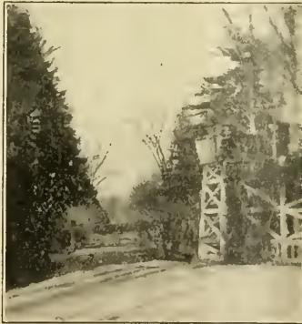
THE AQUEDUCT, CROSSING SUNNYSIDE LANE
