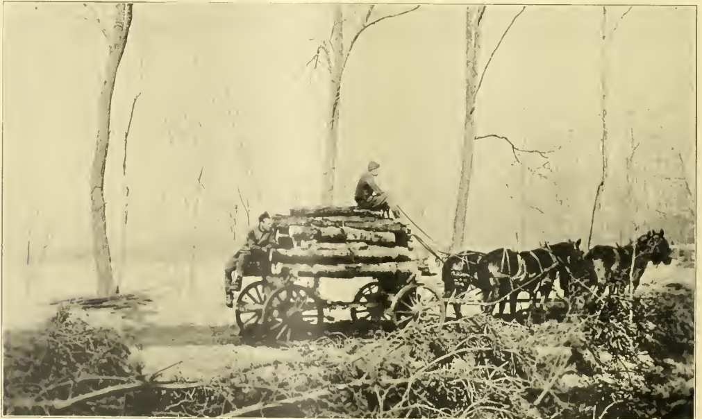
A LOADED AMERICAN LOG WAGON ON ITS WAY FROM THE FOREST IN FRANCE TO A 20th REGIMENT SAWMILL
