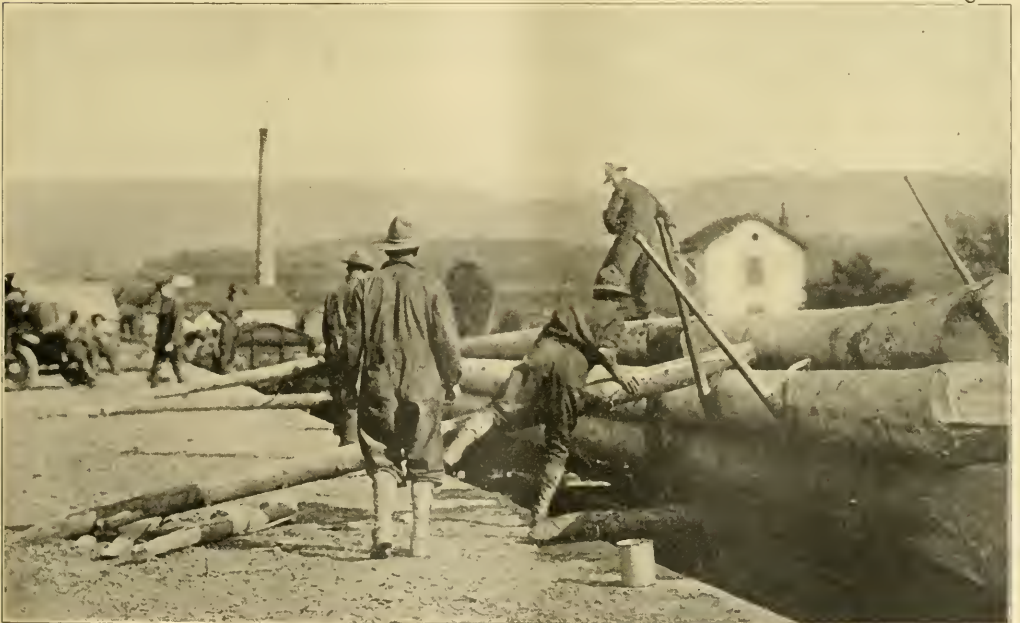
20th ENGINEERS LOADING LONG PILING FOR SHIPMENT FROM EASTERN FRANCE TO BASE PORTS ON ATLANTIC COAST TO BE USED IN DOCK CONSTRUCTION
