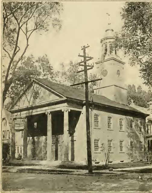
THE EXTERIOR OF THE BUILDING
