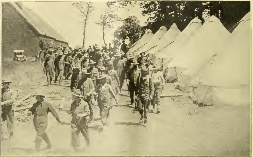
CAMP OF DETACHMENT OF 20th ENGINEERS IN FRANCE. CREW STARTING TO WORK
