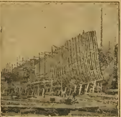
Paying surfaces of timbers brush-treated with Carbosota. (Gardner Peninsula Ship Bldg. Co.)
