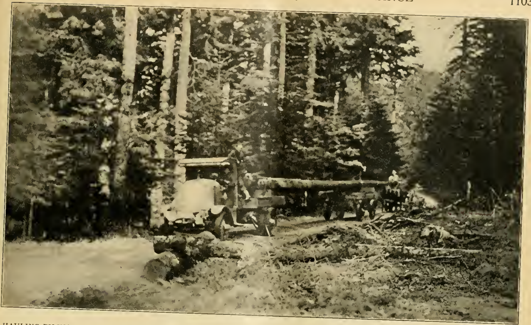
HAULING PILING 60 TO 80 FEET LONG BY MEANS OF MACK TRUCK AND TRAILER FROM THE FOREST TO THE SHIPPING POINT IN EASTERN FRANCE
