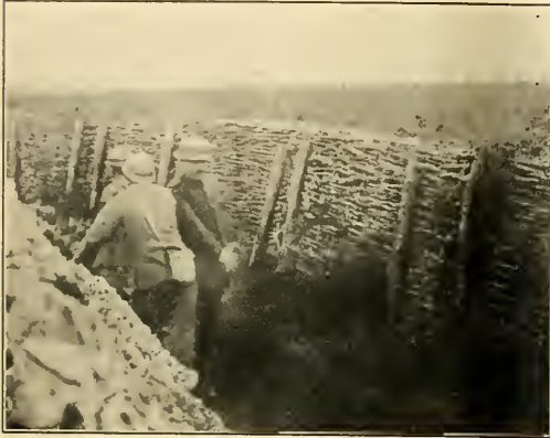
BRUSH FROM FRENCH FORESTS USED IN REVETTING TRENCHES
