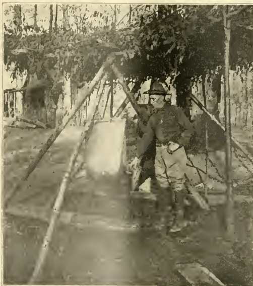
AN AMERICAN FORESTRY ENGINEER AT THE WATER BAG WHICH CONTAINS THE CAMP'S SUPPLY OF DRINKING WATER. THE ROOF OVERHEAD KEEPS THE SUN OFF THE BAG, AND A DITCH CARRIES AWAY THE LEAKAGE
