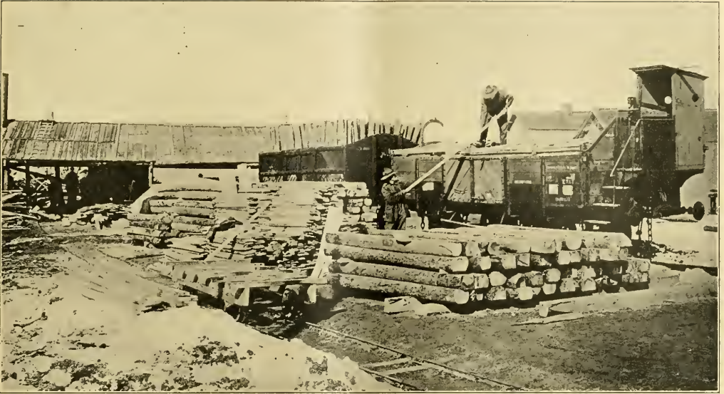
20th ENGINEERS LOADING LUMBER AND TIES ON FRENCH CARS. THE CAR AT THE LEFT IS LOADED WITH BARBED WIRE STAKES. THE BUILDING AT THE END OF THE RIGHT-HAND CAR CORRESPONDS TO AN AMERICAN CABOOSE
