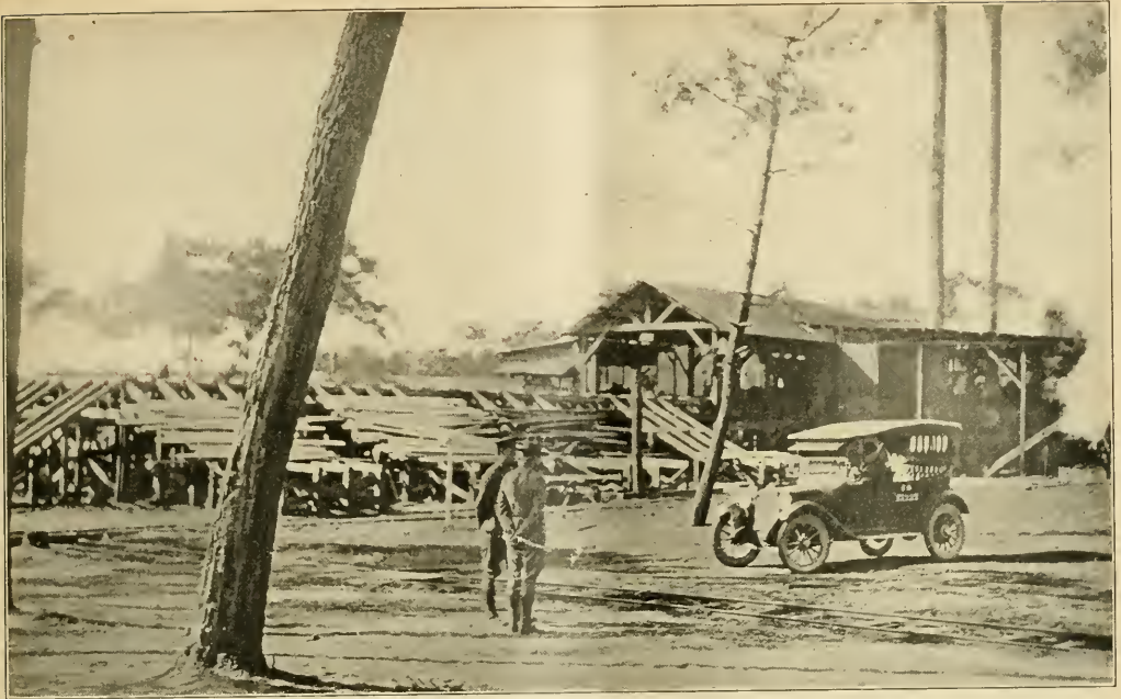
AMERICAN 20-M SAWMILL NEAR PONTENX, LANDES. COL. BENEDICT WITH HIS BACK TURNED, IN THE FOREGROUND, STANDING NEAR NARROW GAUGE TRACK OVER WHICH LUMBER IS TRANSPORTED THREE MILES TO THE SHIPPING YARD
