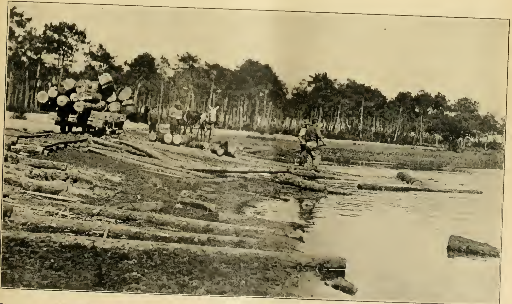
CAR LOAD OF MARITIME PINE LOGS BEING DUMPED INTO AUREILHAN LAKE TO BE TOWED TO THE AUREILHAN AMERICAN SAWMILL NEAR PONTENX, LANDES. NARROW GAUGE RAILWAY SHOWN. THE MULES BRING THE LOGS FROM THE PINE FORESTS OF THE SAND DUNES.
