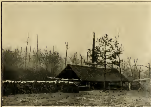
A TYPICAL MOUNTAIN STAVE MILL
