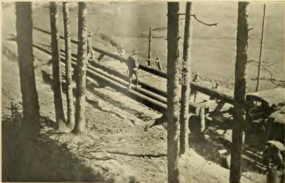
MEMBERS OF THE 20th ENGINEERS LOADING PILING ON TRUCKS AT LANDING No. 2 IN FRANCE. THESE PILINGS ARE APPROXIMATELY SEVENTY FEET LONG
