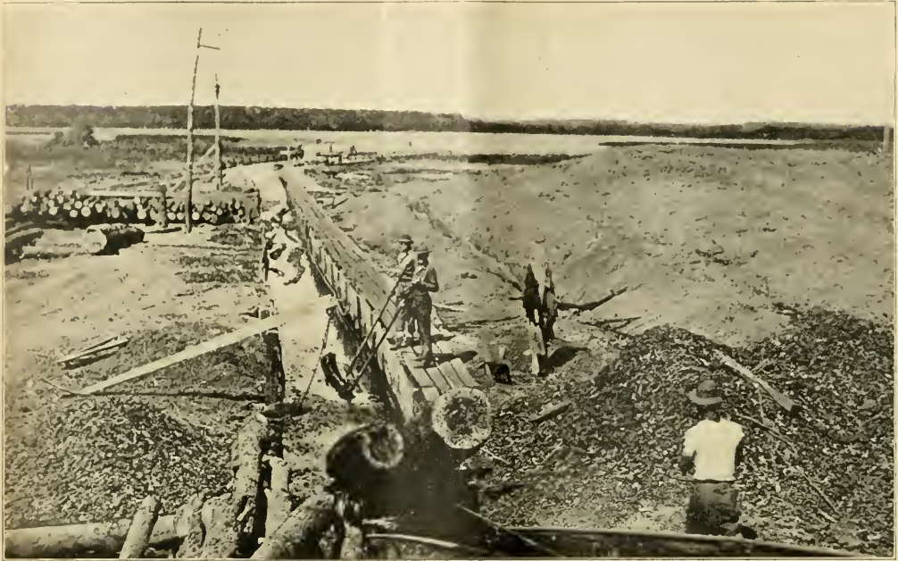
VIEW OF AUREILHAN LAKE, FRANCE, FROM AMERICAN 20-M SAWMILL. LOGS WERE TOWED ACROSS THE LAKE FROM THE MOUTH OF THE COURANT RIVER, BROUGHT TO THE BOOMS AT THE EDGE OF THE LAKE, THEN POLED ALONG THE CANAL TO THE POINT IN THE FOREGROUND WHERE THEY WERE LOADED UPON A SMALL CAR WHICH WAS PULLED BY CABLE UP THE INCLINE INTO THE SAWMILL. THE LARGE HEAP OF SAWDUST AT THE RIGHT WAS PRODUCED BY THE MILL AS THE RESULT OF SEVERAL MONTHS' OPERATION
