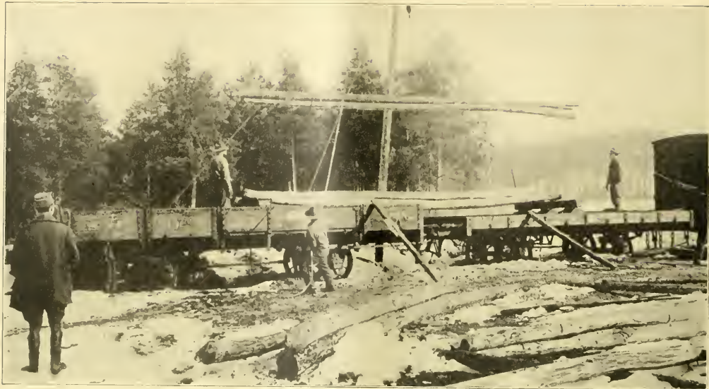
LOADING PEELED POLES ON TO RAILWAY CARS AT ONE OF THE OPERATIONS OF THE 20th ENGINEERS
