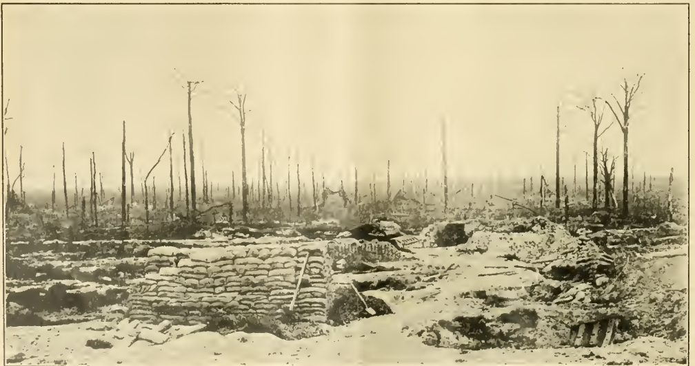
A SCENE IN THE BOIS DES LUPINS NEAR BOESINGHE, SHOWING THE GERMAN FORTIFICATIONS AND THE DESTRUCTION DONE TO TREES AND FORTIFICATIONS BY SHELL FIRE.
