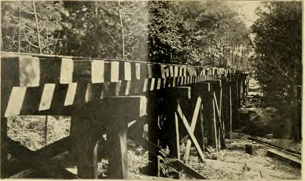
PORTIONS OF TRESTLE BUILT BY THE 20th ENGINEERS IN THE MARITIME PINE FOREST IN THE LANDES, IN SOUTHWESTERN FRANCE TO TRANSPORT FOREST PRODUCTS FROM THE WOODS TO THE MAIN LINE
