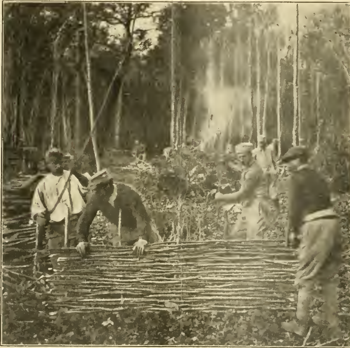
WEAVING SUPPORTS FOR SIDES OF TRENCHES
