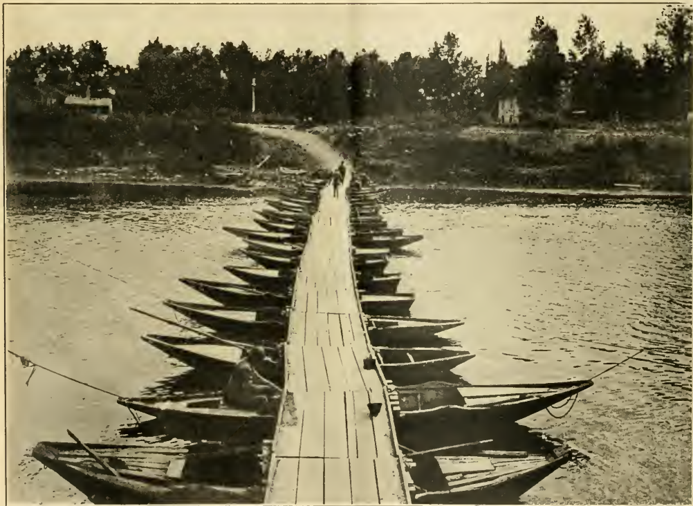
A PONTOON BRIDGE ACROSS THE MARNE
