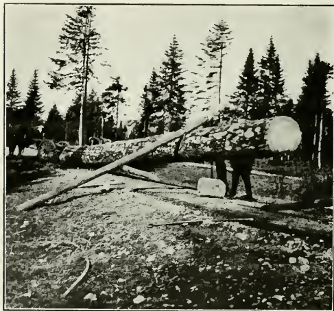
A NOVEL ONE-MAN METHOD OF LOADING A TREE. EQUIPMENT USED: A POLE, TWO CHAINS, A BLOCK OF TIMBER AND A POWERFUL JACK
