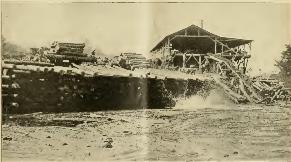
MARITIME PINE LOGS BEING UNLOADED FROM NARROW GAUGE CARS INTO MILL POND IN PINE FORESTS IN SOUTHWESTERN FRANCE. AMERICAN 20-M MILL IN BACKGROUND
