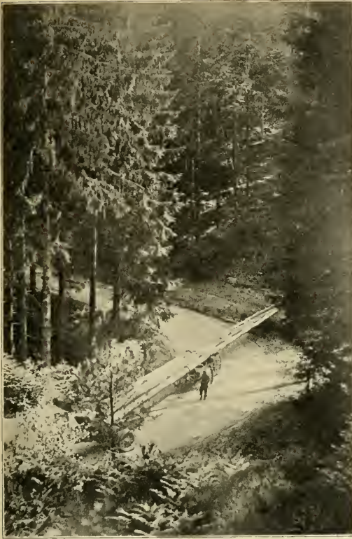
A LOAD OF PILING APPROXIMATELY 70 FEET LONG ON MOTOR TRUCK AND TRAILER GOING AROUND SHARP TURN IN THE ROAD IN A FRENCH SPRUCE FOREST. OPERATIONS OF 20th ENGINEERS
