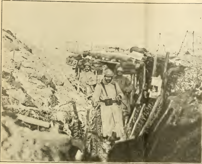
LUMBER USED IN TRENCH CONSTRUCTION
