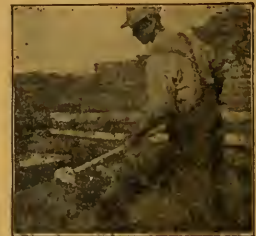
Brush-treating pole. Note use of a mop, which is more satisfactory than a brush.
