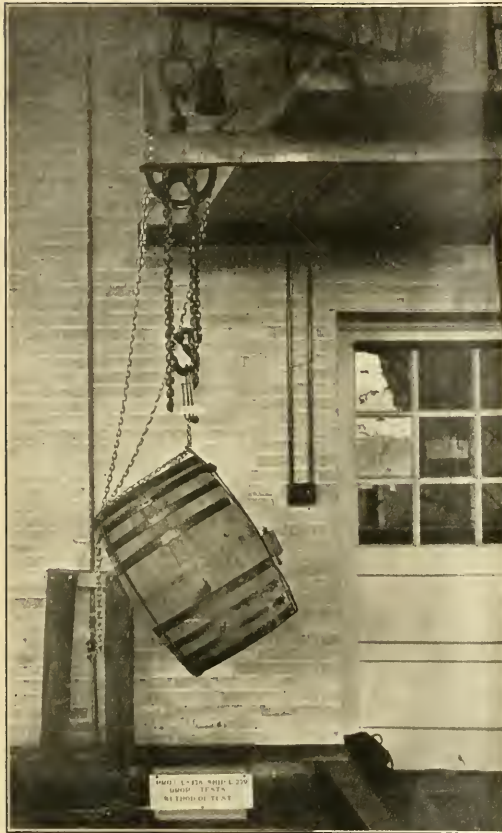
THE CHINE TEST FOR BARRELS
