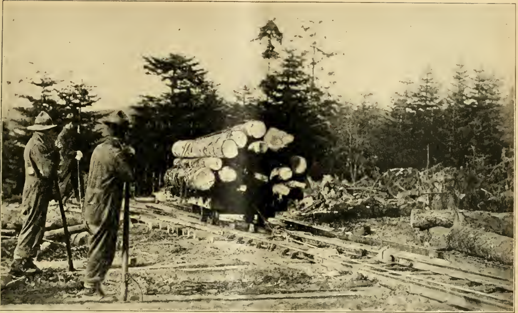
LOAD OF LOGS WHICH HAS JUST BEEN LOWERED DOWN A STEEP INCLINE. THE CABLE BY WHICH THE CAR OF LOGS HAS BEEN LOWERED IS SEEN BETWEEN THE RAILS AT THE RIGHT.
