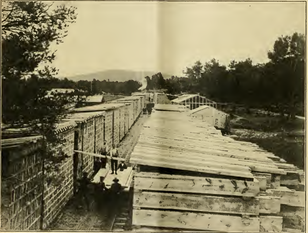
TIMBER STACKS AT A CANADIAN CAMP
