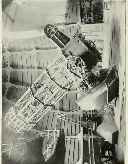
SIXTY-INCH REFLECTING TELESCOPE WITH CASSEGRAIN SPECTOGRAPH IN THE MOUNT WILSON SOLAR OBSERVATORY.
