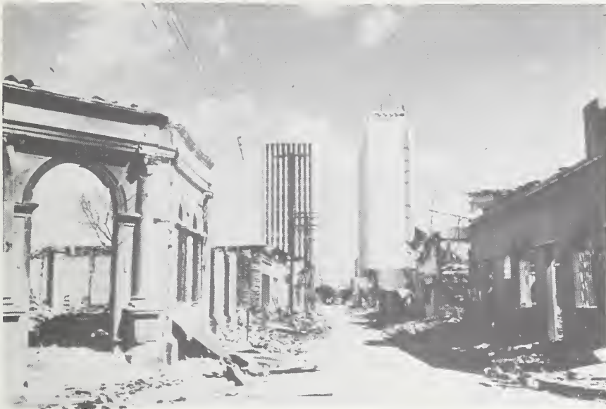
Figure 52-1 Banco de America (left) and Banco Central (right) survived amid collapsed low buildings of taquezal construction.
