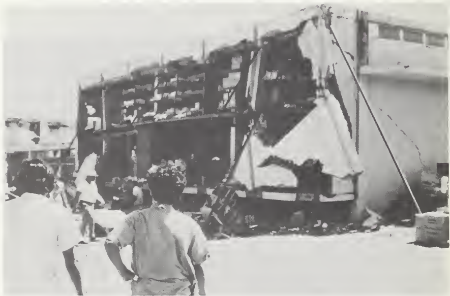
Figure 55-8 Medical supply warehouse supported by shelving inside, Hospital General El Retiro.
