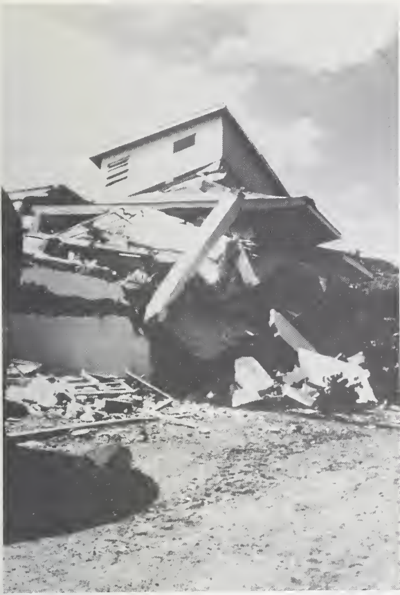
Figure 68-1 View of general collapse, Aduana General de Managua.
