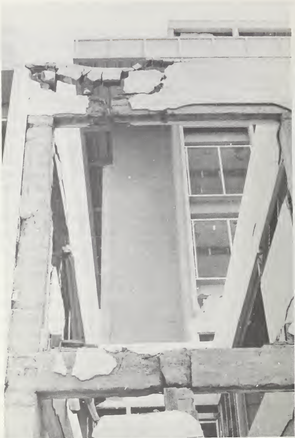
Figure 43-1 Ruptured beams connecting building elements across a courtyard, Corte Suprema de Justicia.
