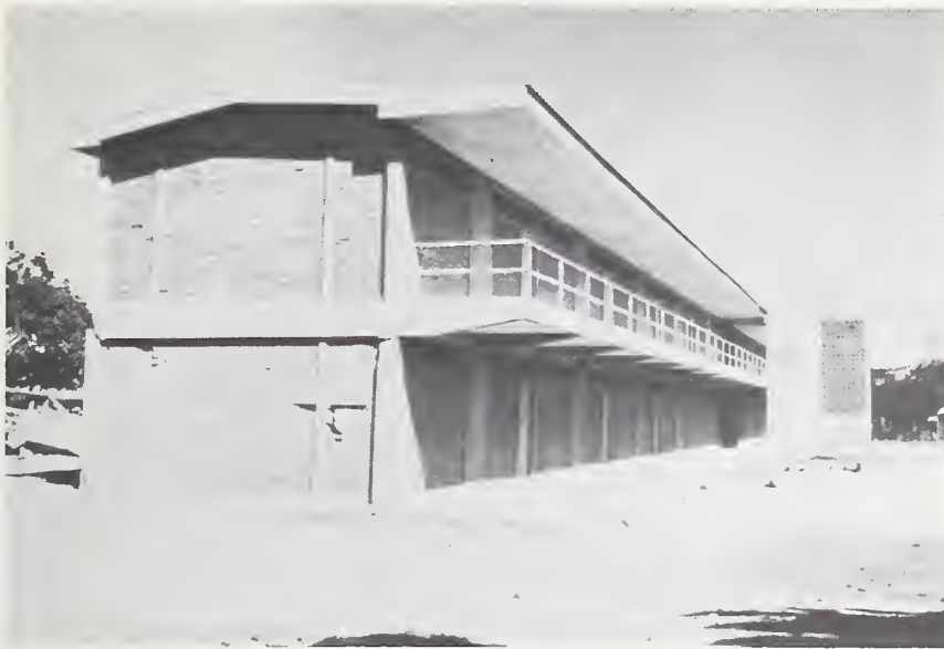
Figure 35-2 New building of reinforced concrete and masonry construction, Centro Escolar Simon Bolivar.
