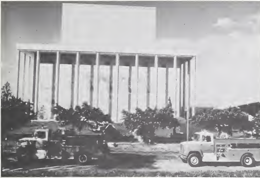
Figure 41-1 South facade of theatre showing some loss of finish, Teatro Ruben Dario.
