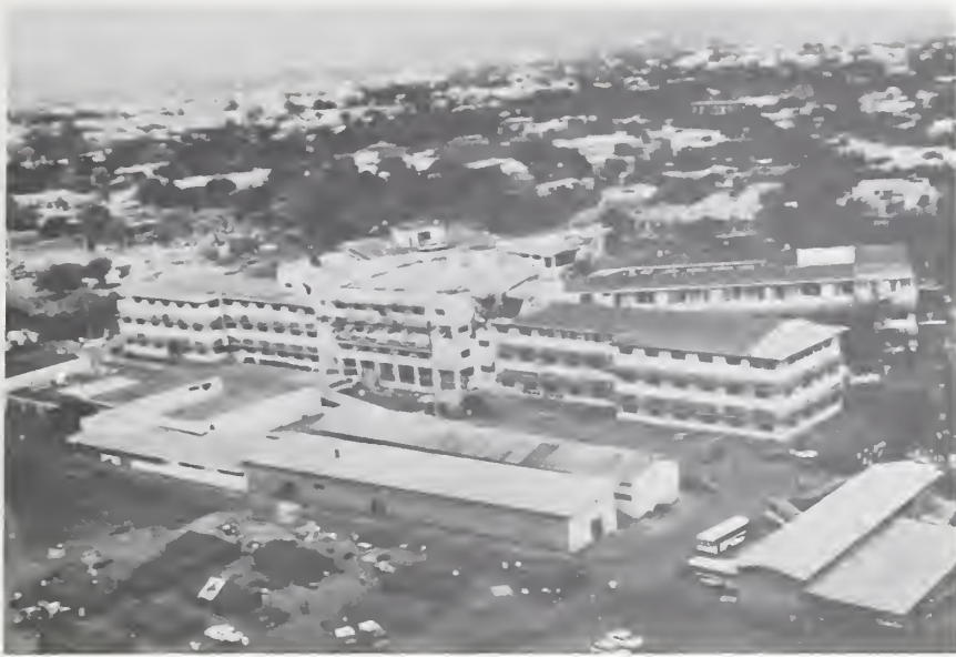
Figure 55-1 Aerial view from the rear, Hospital General El Retiro.
