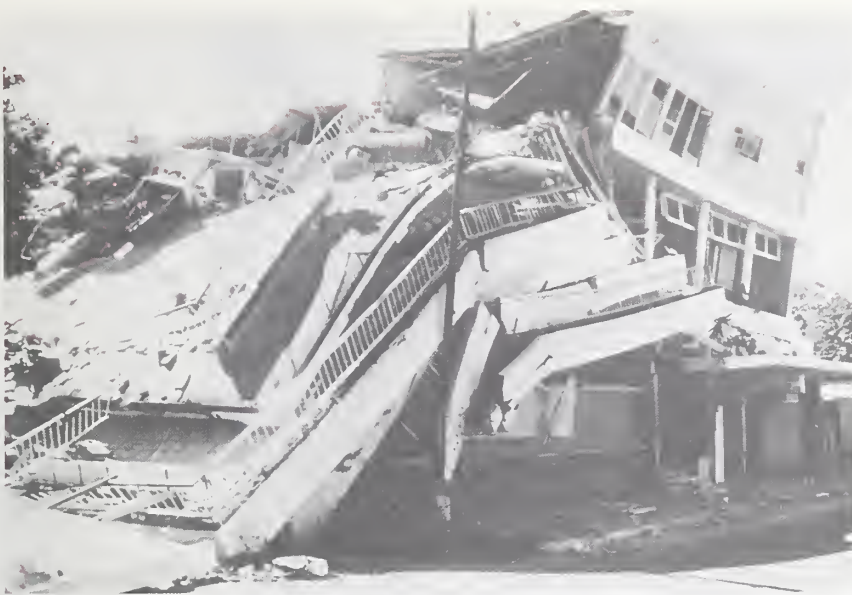
Figure 74-1 Four of five stories collapsed, Edificio Guerrero Pineda.
