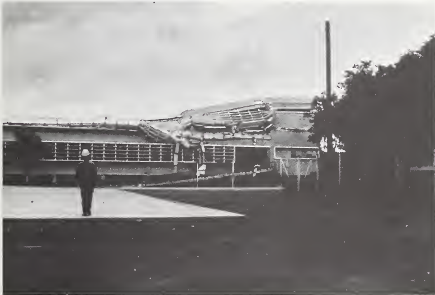
Figure 38-2 Collapse of upper two stories of the west wing from the courtyard, Instituto Nacional Ramirez Goyena.
