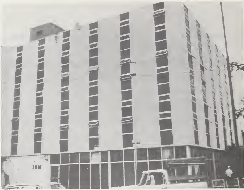
Figure 72-1 General view of IBM building.
