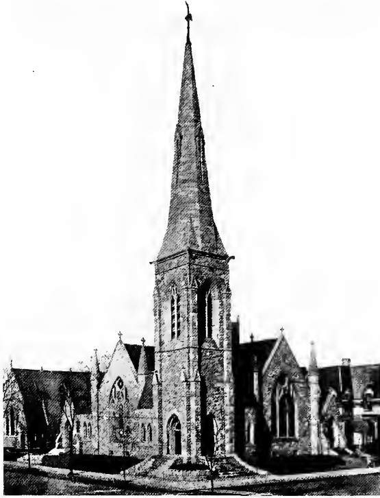
THE NORTH REFORMED CHURCH OF PASSAIC, ---1891.
