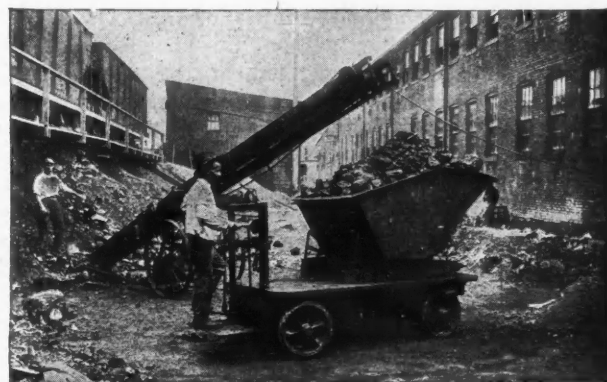
FIG. 2. LOADING ON A STORAGE-BATTERY TRUCK
