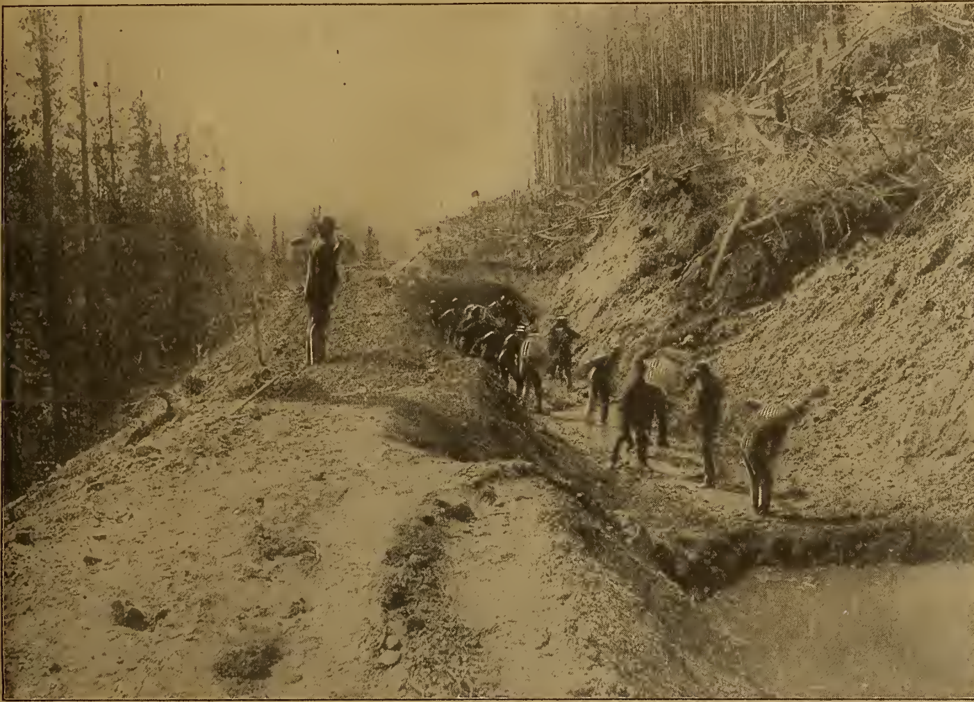
CLEANING OUT AN EARTH-SLIDE IN THE BIG LARAMIE DITCH
