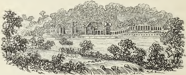
[Fig. 250. View of Endsleigh Cottage, on the banks of the Tamar.]
