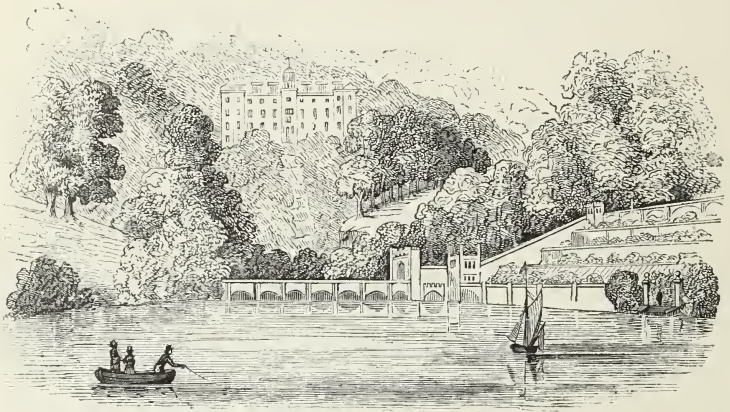
[Fig. 179. View of Beaudesert as it will appear when the woods are opened and other improvements effected.]
