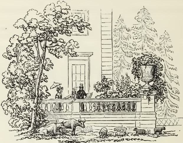
[Fig. 159 Terrace fence, separating the Italian garden from the park.]
