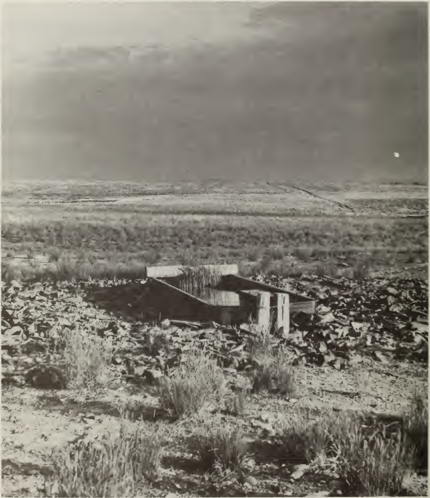
Fig. 17. A trough receiving water from a pipeline for the use of livestock and wildlife. (Photo by author)
