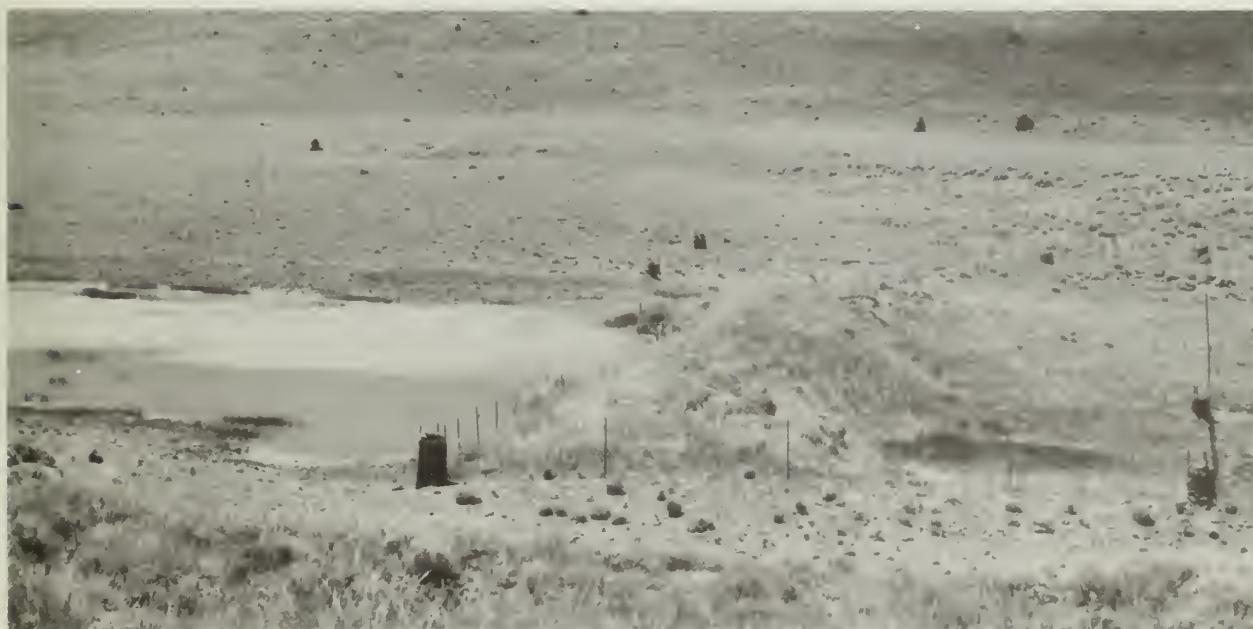
Fig. 11. A small reservoir, with a fence to protect vegetation on the dam, constructed for pronghorns and livestock on the Hart Mountain National Wildlife Refuge, Oregon. (Photo by author)
