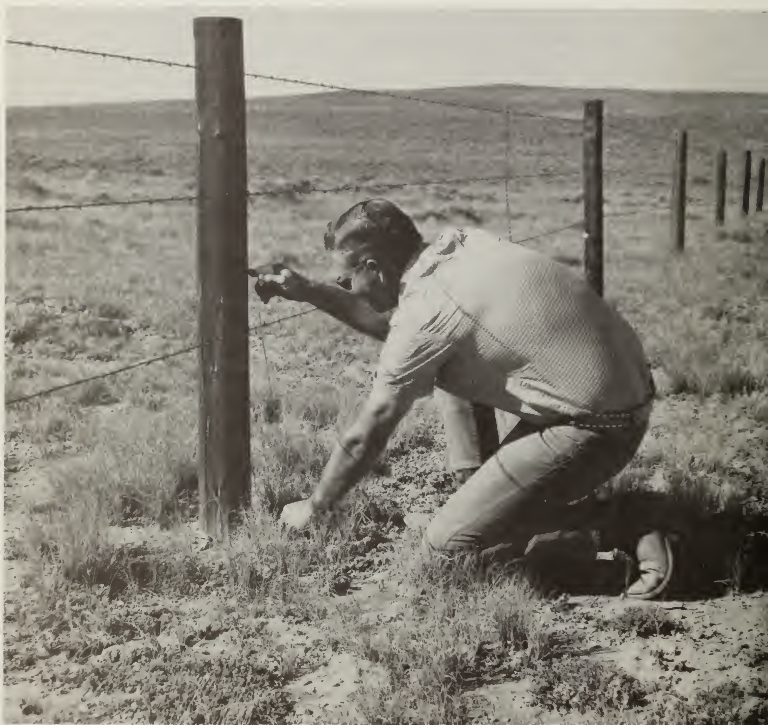
Fig. 19. Checking a barb wire fence to make sure the bottom wire meets requirements of 16" from the ground for pronghorns. (Photo by author)
