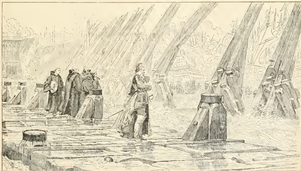
RICHELIEU SURVEYING THE WORKS AT ROCHELLE.
