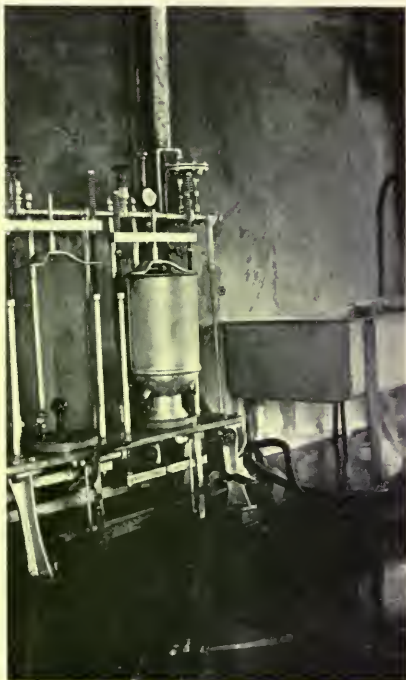
Fig. 151.—Steam sterilizer for cans.
