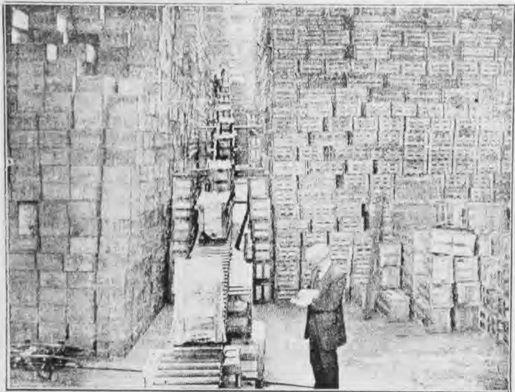
FIG. 61.—Gravity runway at Trafford Park warehouses, Manchester. (W. & C. Panton.)
