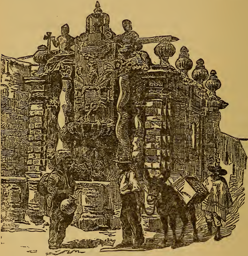
TERMINATION OF AQUEDUCT.
