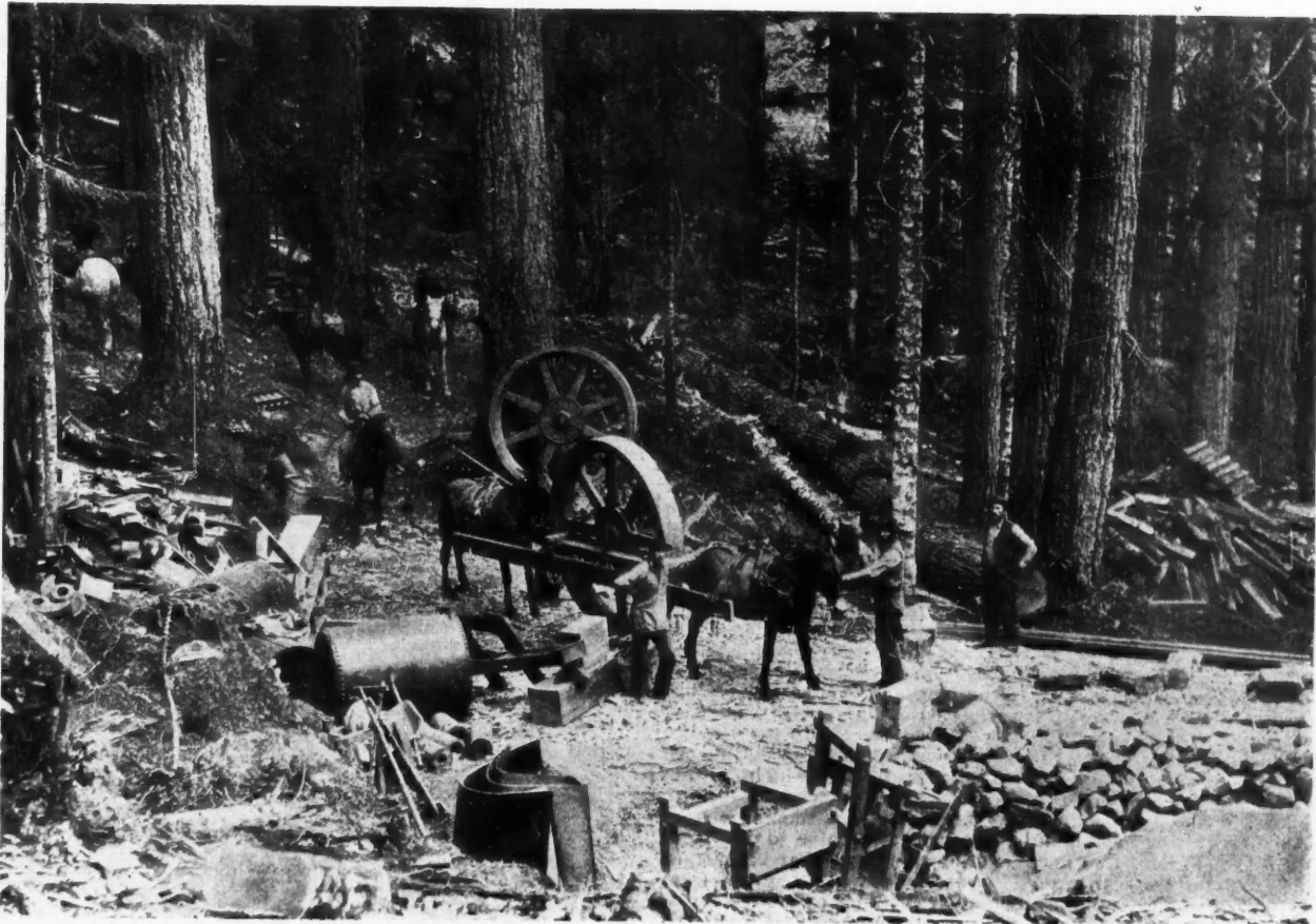
PACKING CAM SHAFT PULLEY, 7 FT. DIAMETER.
