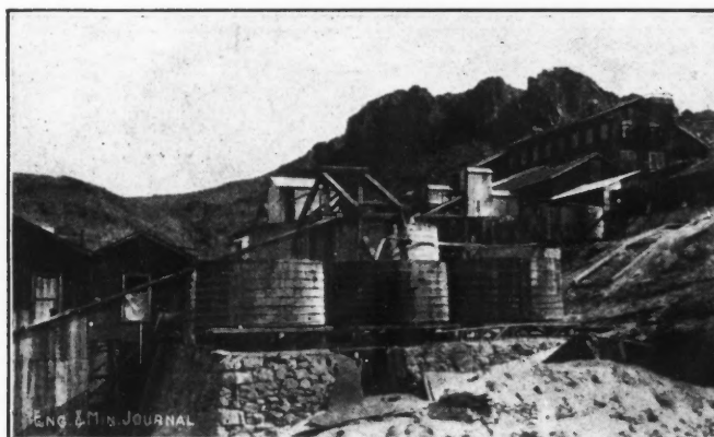
LOOKING TOWARD THE CRUSHING PLANT GOLD ROAD MILL,
