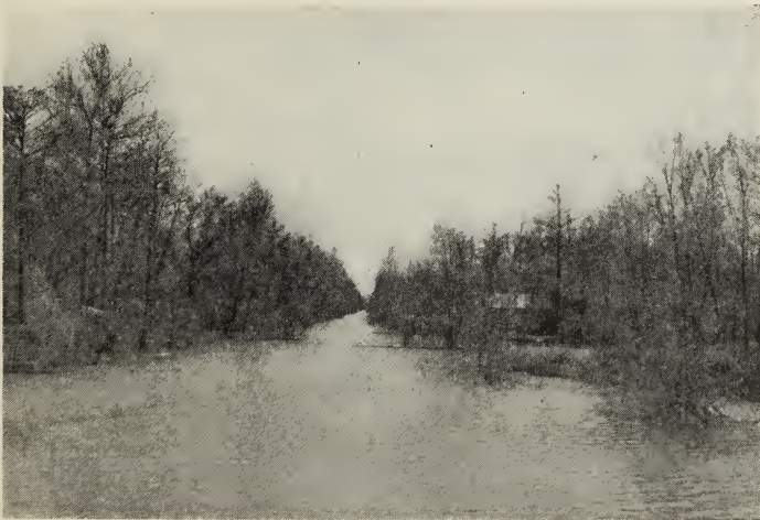
Figure 1. The Spillway, Reelfoot Lake, Tennessee. April 9, 1939. At high water stage.
