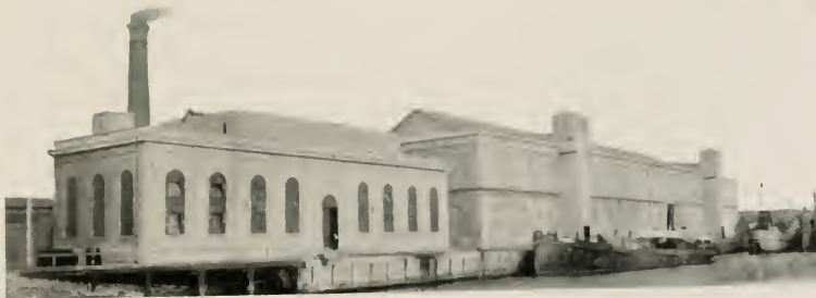
THE NEW COLD STORE AT SOUTHAMPTON DOCKS, L. AND S. W. R. (Leased to the International Cold Storage and Lairage Co. Ltd.)
