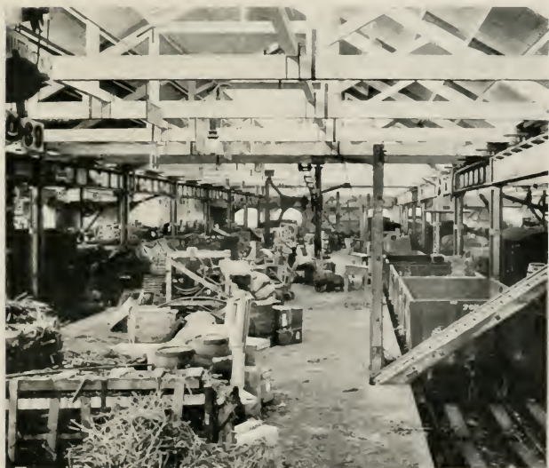
INTERIOR OF GOODS TRANSHP SHED, CREWE, L. AND N. W. R.
