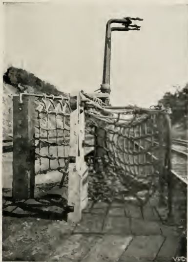
APPARATUS FOR RECEIVING AND DELIVERING MAIL-BAGS TO AND FROM A TRAIN IN MOTION. The bag drops into an elastic net carefully adjusted to take off the force of the impact.
