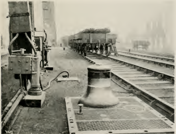
ELECTRIC CAPSTAN FOR SHUNTING WAGONS AT MIDDLESBROUGH DOCKS, N. E. R.
