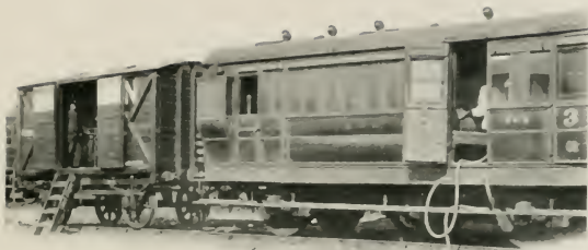
VACUUM-CLEANER IN USE FOR RAILWAY CARRIAGES, G. N. R.
