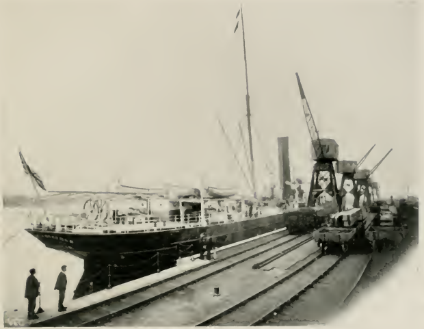
ELECTRIC TRAVELLING CRANES AT MIDDLESBROUGH DOCKS, N. E. R. Photo by M. Wright.]
