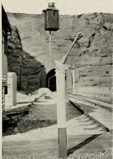
APPARATUS FOR SINGLE-LINE WORKING, G. W. R. The "staff," with looped handle, in position to be picked up by driver of a train passing at speed.
