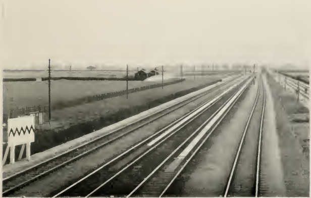
"PICK-UP" WATER-TROUGHS NEAR PETERBOROUGH, G. N. R.
