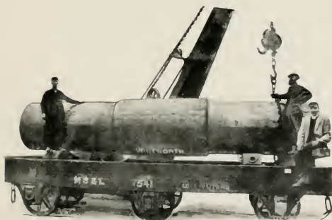
GUN-COIL LOADED ON M S. AND L R. WAGON.
