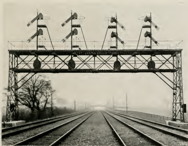
FOUR-TRACK AUTOMATIC SIGNAL GANTRY, L. AND S. W. R.
