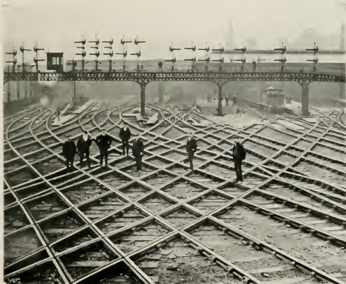
APPROACH TO NEWCASTLE CENTRAL STATION, N. E. R.
