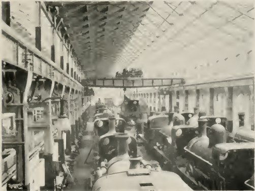
ELECTRIC TRAVELLING CRANE IN LOCOMOTIVE-REPAIRING-SHOP, DONCASTER, GREAT NORTHERN RAILWAY.
