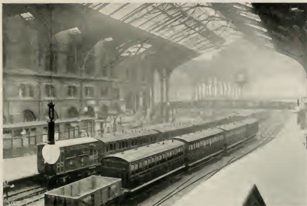
PART OF THE INTERIOR OF LIVERPOOL STREET STATION, LONDON, G. E. R. Photo by the Locomotive Publishing Company.]
