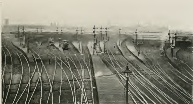
ENTRANCE TO WATERLOO STATION, L. AND S. W. R.
