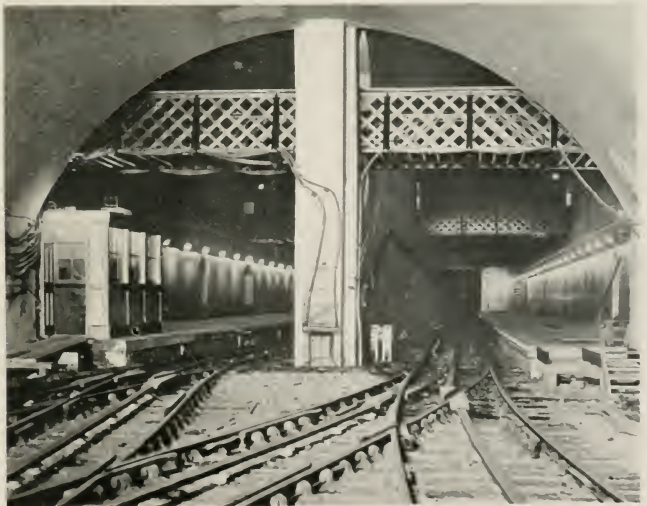
WATERLOO TERMINUS, WATERLOO AND CITY ELECTRIC RAILWAY.
