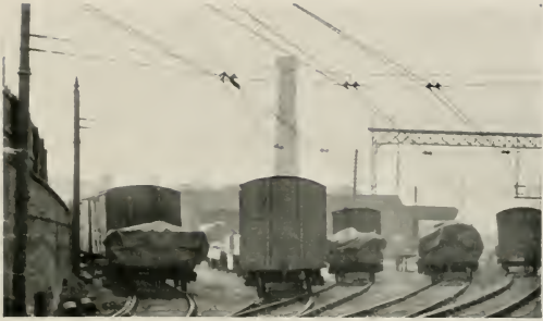
OVERHEAD CONSTRUCTION FOR WORKING GOODS TRAFFIC BY ELECTRICITY. MANORS (NEWCASTLE) GOODS YARD, N. E. R.
