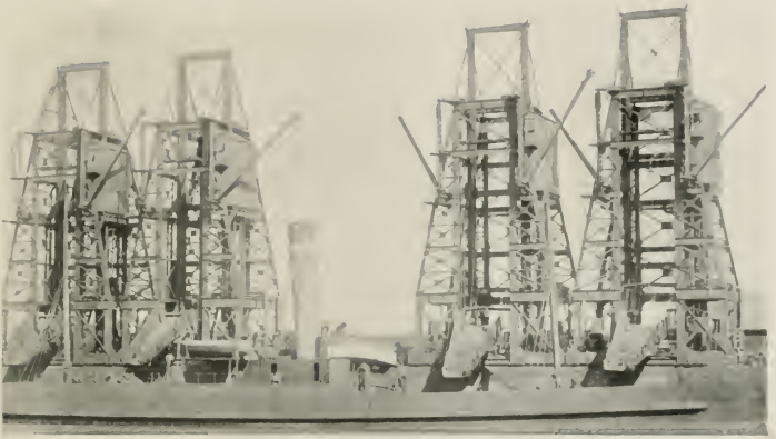
THE FOUR MOVABLE HYDRAULIC COAL-TIPS AT PENARTH DOCK, TAFF VALE RAILWAY.
