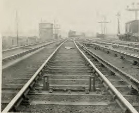
TRAIN-STOPPING APPLIANCE. THE APPARATUS IN POSITION PARTIALLY TO APPLY THE BRAKES OF AN APPROACHING TRAIN, N. E. R.
