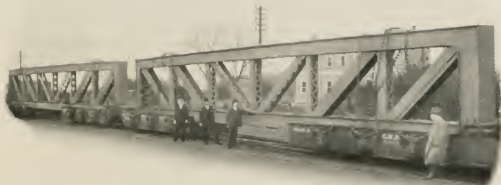
TWO LARGE GIRDERS LOADED ON G. W. R. TROLLEY-WAGONS.
