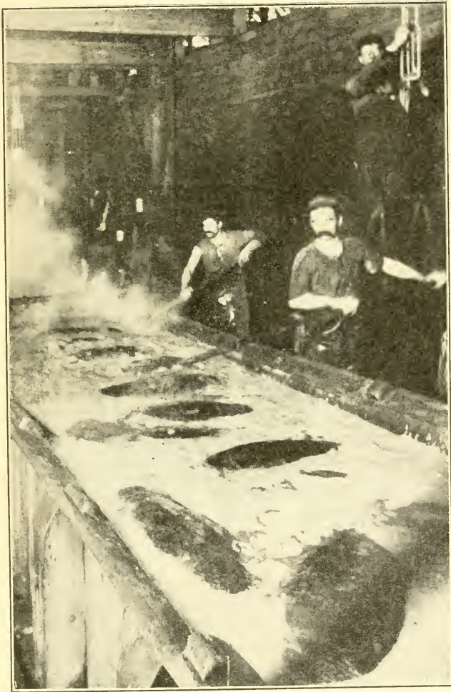
On the way to the scraper—Hog scalding vat. The temperature of the water is kept at about 150° Fahr.
