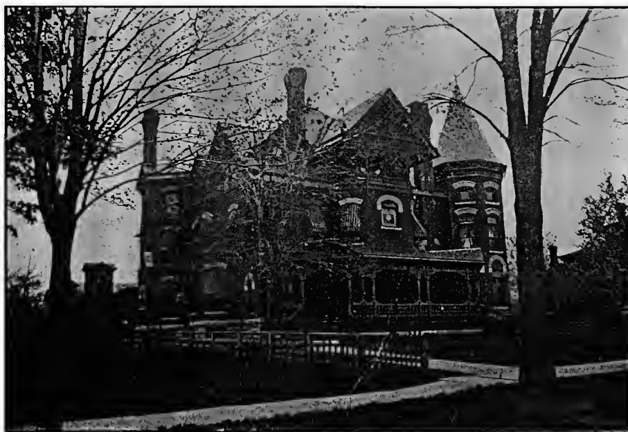
SEABURY S. GOULD'S RESIDENCE.
