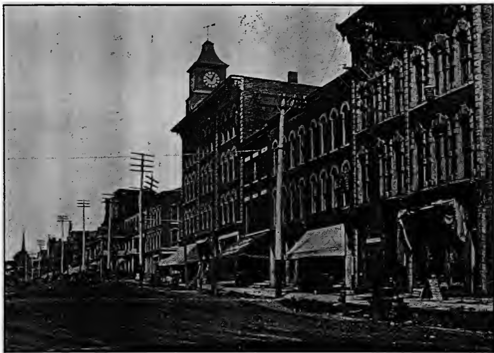
Pruden, Photo. FALL STREET, NORTH SIDE, LOOKING WEST FROM OVID STREET.
