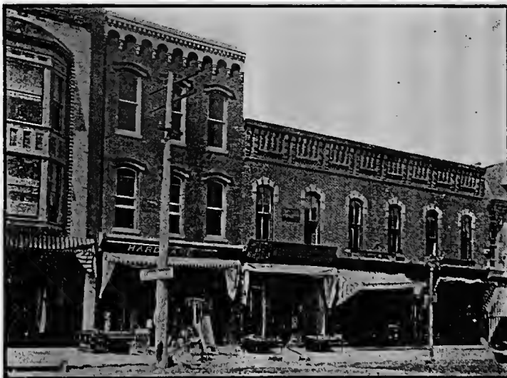
FAILING BUILDING. MILLER BLOCK, 106-112 Fall Street.
