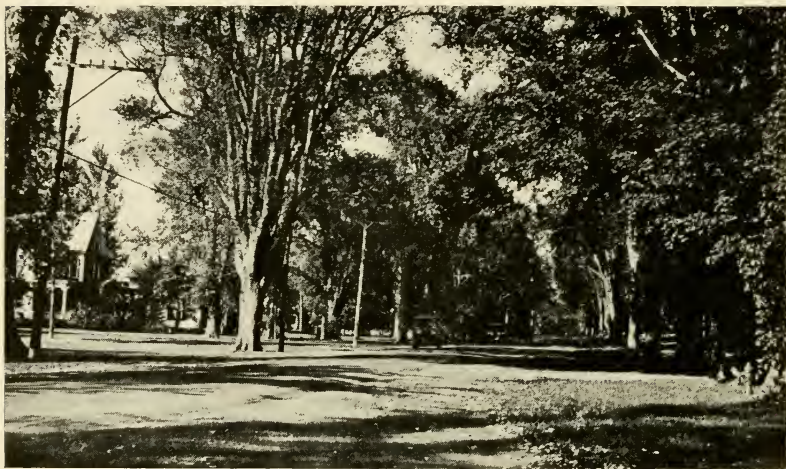
Main Street, 1923, looking north from near the Belcher Fountain
