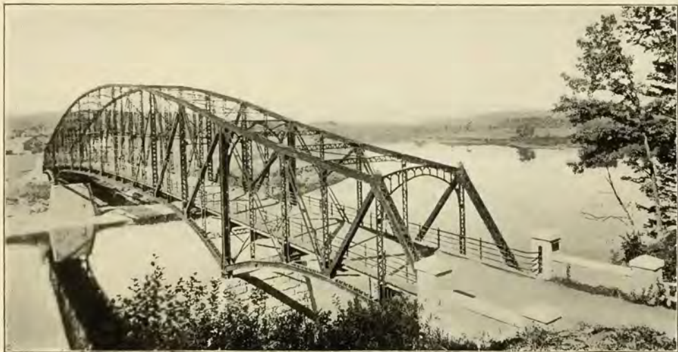
Schell Bridge, crossing the Connecticut River between East and West Northfield, erected in 1903 in memory of Robert and Mary Schell of New York by their son, Francis Robert Schell
