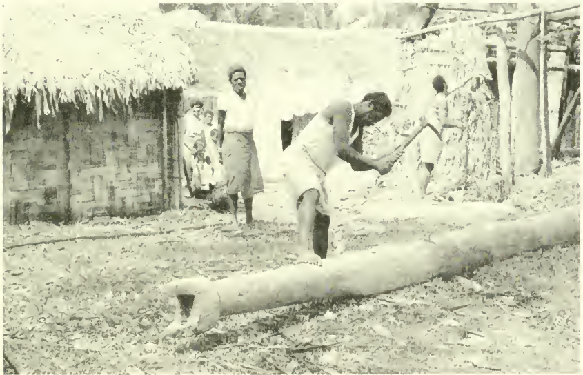
2. An upright for a house is shaped from a tree trunk with an adz. The usual tools for house building in Fiji are the machete, ax, and adz.
