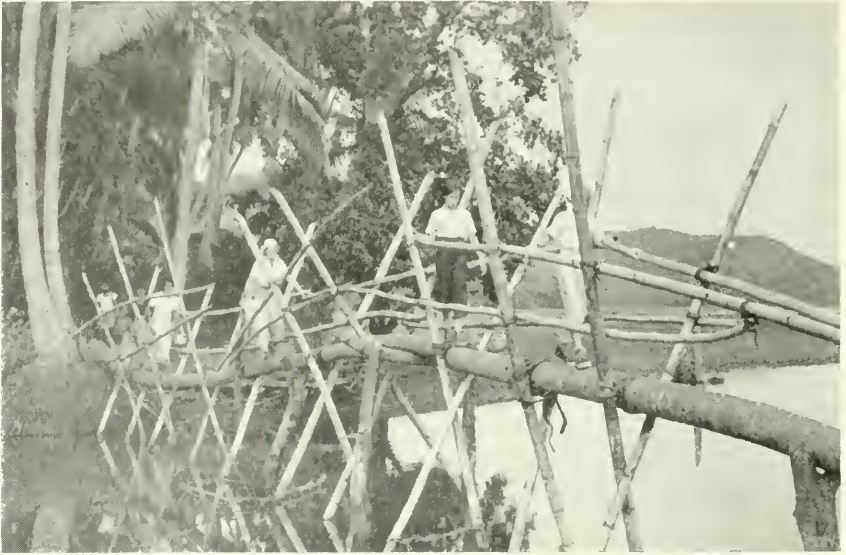
1. A footbridge of palm trunks and bamboo stems crosses a tidal creek on Ngau. The Fijians are adept builders with local materials, and such a temporary fiber-lashed structure is made in a matter of minutes.
