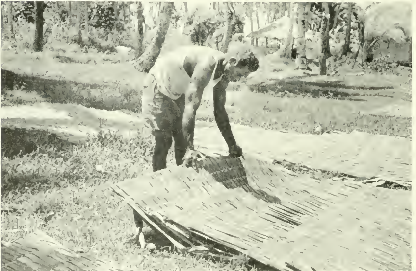
2. The leaf segments of Metroxylon vitiense are taken from the leaves, bent around a reed, and sewed together with hibiscus fiber. "Shingles" about six feet long are dried in the sun and then tied to the rafters of the roof. Such thatching is said to be durable for 20 years or more.
