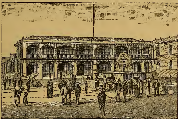
The Government Building, Quezaltenango.
