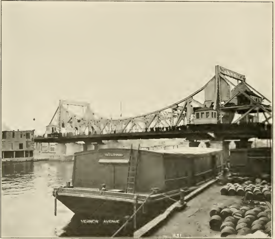
VERNON AVENUE BRIDGE OVER NEWTOWN CREEK.
