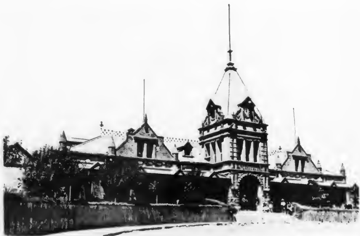
STATION OF THE INTEROCEANIC RAILWAY.
