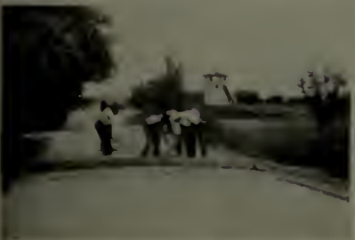
Spreading the stone for the wearing-course
