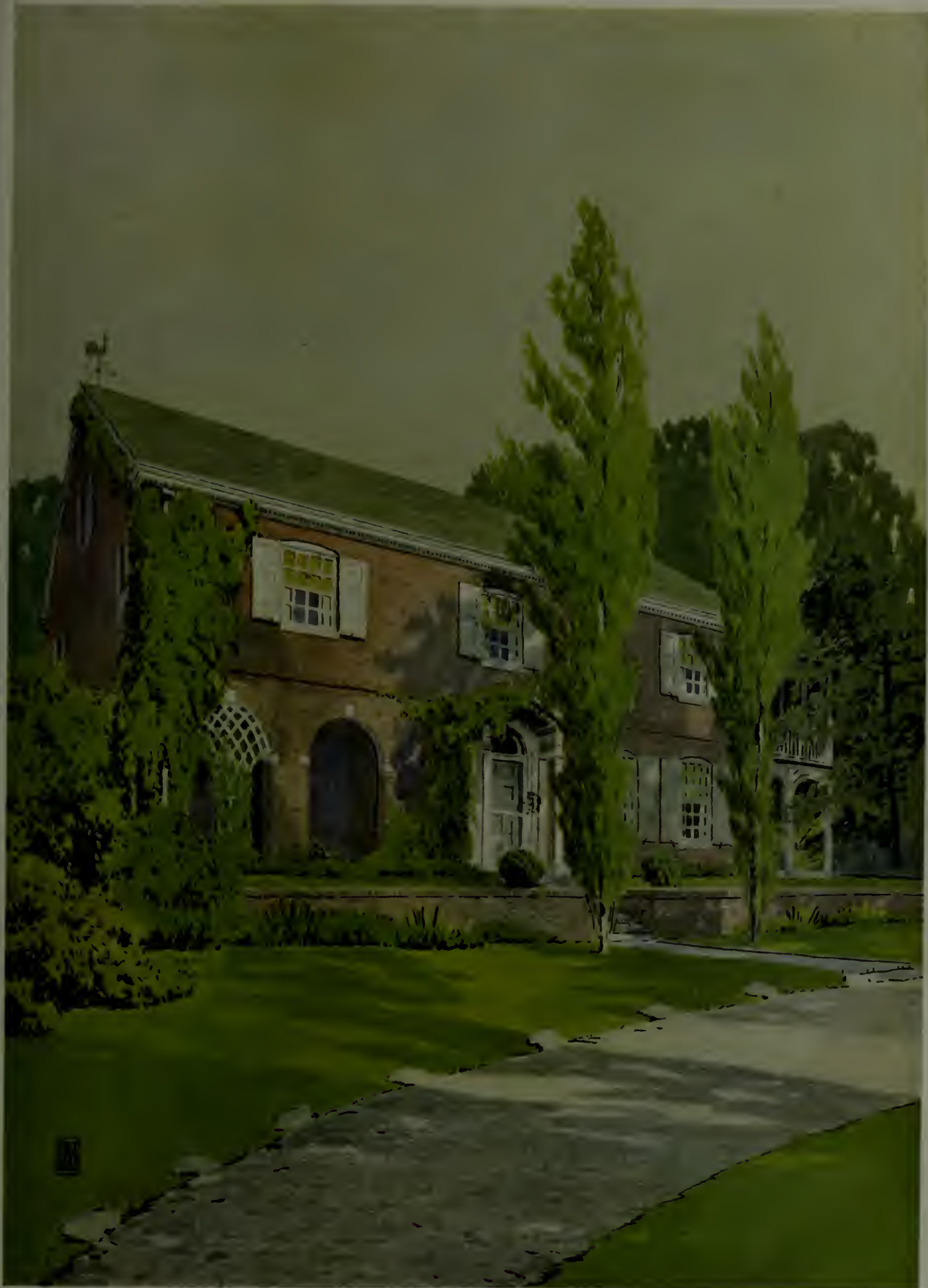
The house of Mr. Pierre Jay Wurts, Englewood, N. J. There are many opportunities for variation in color of the brick house, made possible through modern brick of varied texture, form, and color, but usually only a white—or possibly a dark—trim and a green roof may be used to best advantage
