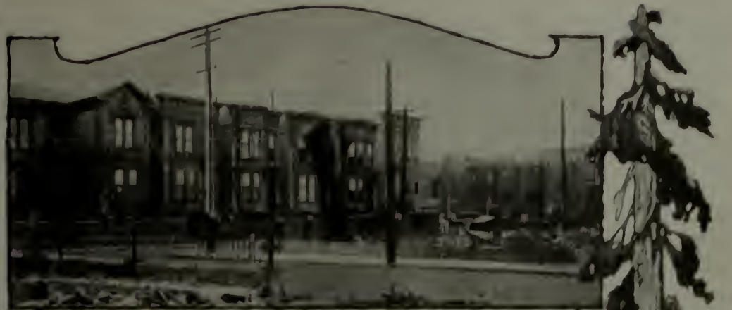
The big San Francisco fire of 1906 was stopped in many places where Redwood buildings faced the conflagration—as shown by these Redwood frame dwellings at 20th and Mission streets, which were scorched but refused to burn. The telephone poles are also Redwood.
