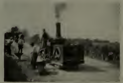
Rolling the three-quarter inch stone into the first coat of Tarvia
