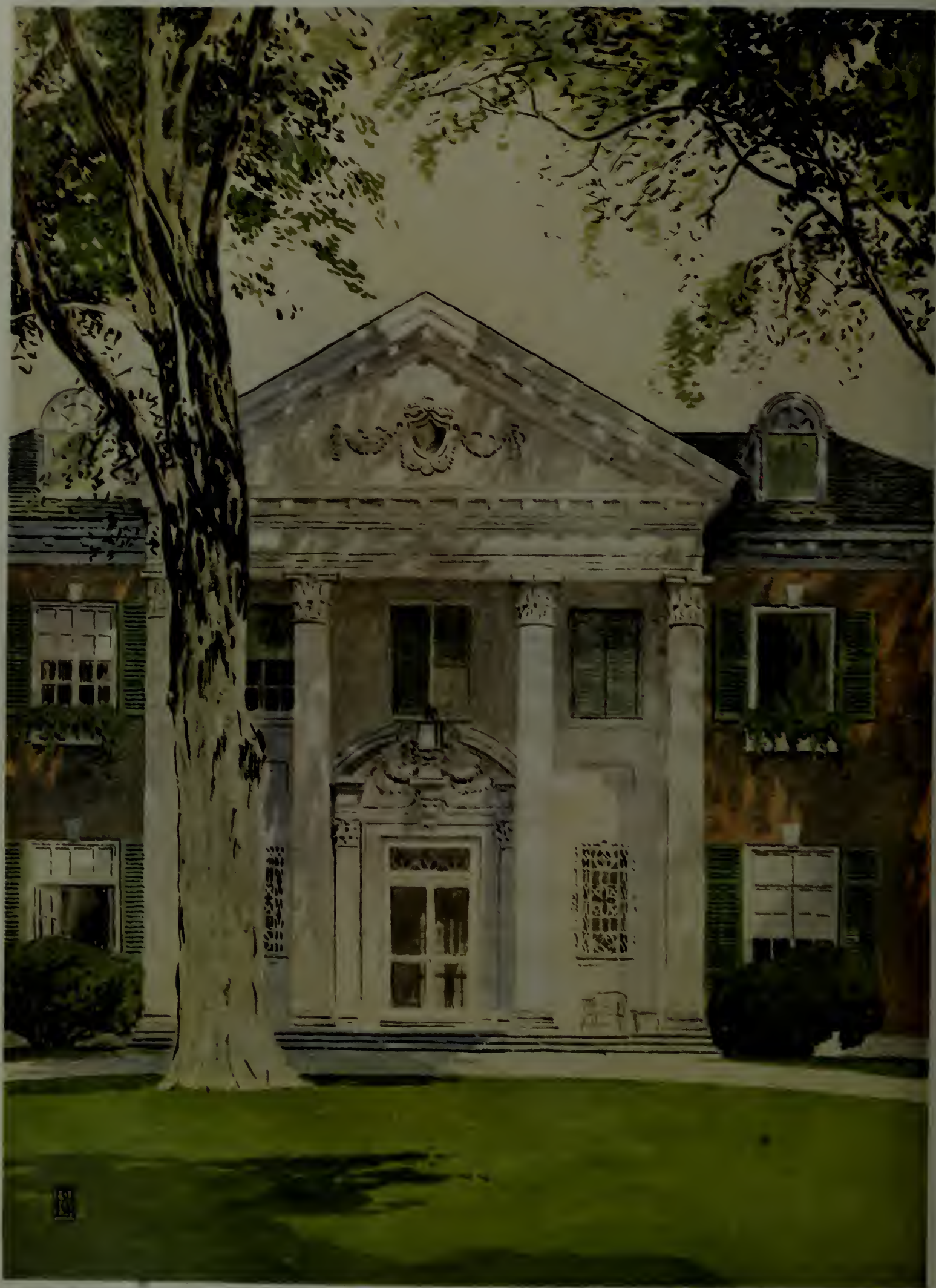
The home of Mr. John T. Pratt, Glen Cove, L. I., is an example of the traditional combination of brickwork with limestone which carries out the stately dignity of the Georgian house. White trim with green blinds and slate roof form the natural accompaniment
