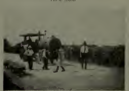
Putting on seal-coat of Tarvia
