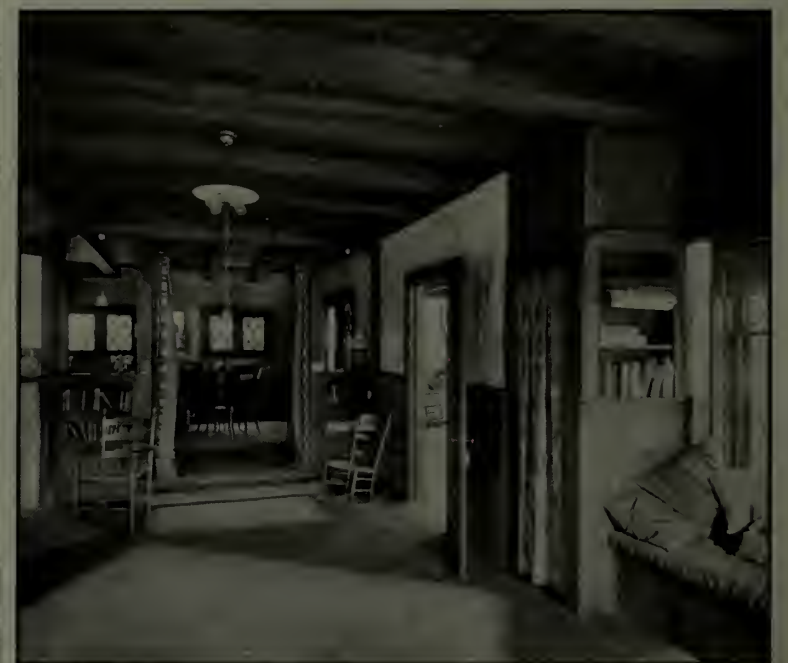
The half partitions between the living and dining rooms give some seclusion without making it impossible to use the two as one room
