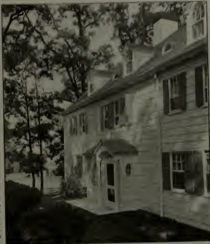
Close up of the new entrance to the Brown house, showing also the dormers which have replaced the one out-of-scale central window.
