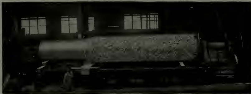
Indiana Limestone column over 30 feet long and 4 feet in diameter being turned on a lathe.
