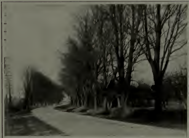
The concrete on the Olcott-Lockport Road, Niagara County, N. Y., is one of the many examples of this durable construction in New York State. Built by the State Highway Department, Edwin Duffey, Commissioner; H. M. Cowles, Rochester, N. Y., Contractor.
