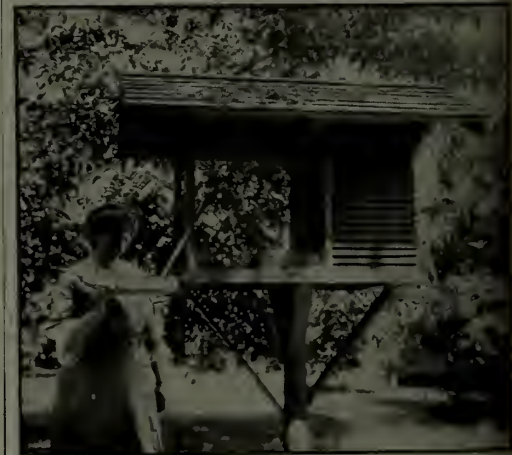
Side view, showing open-air compartment
