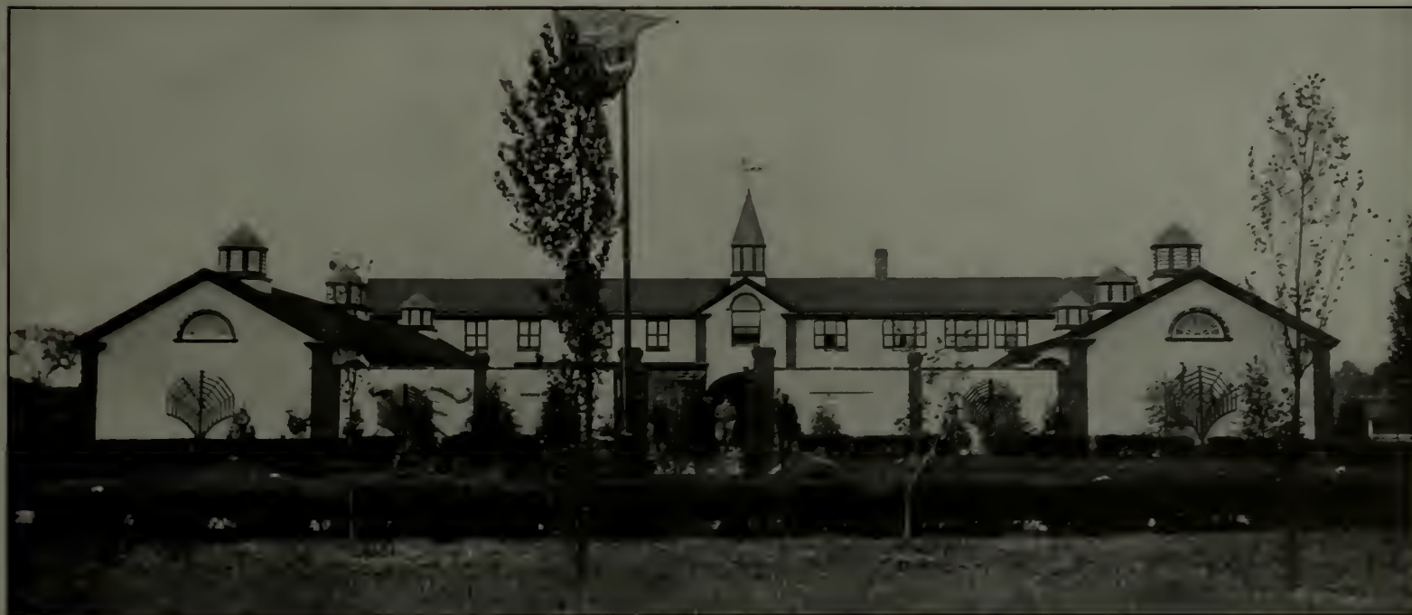
Mr. J. B. Thomas's kennel building, the home of the Piedmont foxhounds and beagles. The length of the main structure is 125 feet; of the wings (which form a court as shown above) 110 feet. Under the one roof are huntsman's living quarters, hound cook room, hound feeding room, courts before and after feeding, wash room, store rooms, hospital, lodging rooms, and whelping rooms and courts. The kennel accommodates seventy-five couples of foxhounds and beagles.
