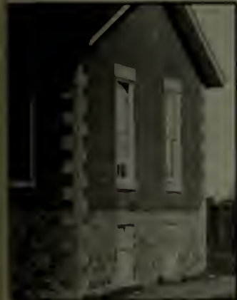
Showing corner construction of school-house, Gypson, N. Y.
