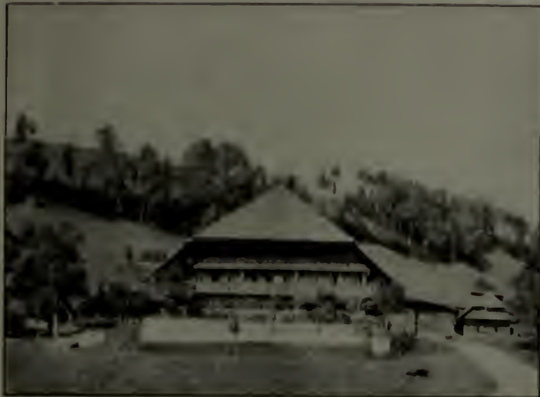
A typical large Swiss farmhouse. Note the roof sheltering the driveway.
