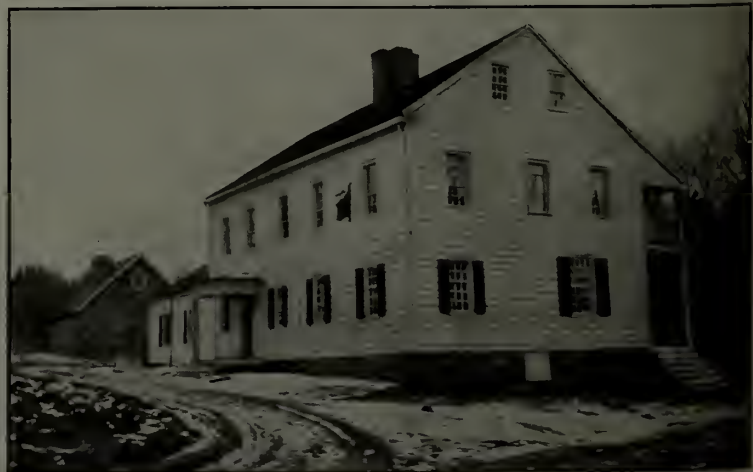
The present front, with the new road passing the door. The stone building at the left is the separate kitchen
