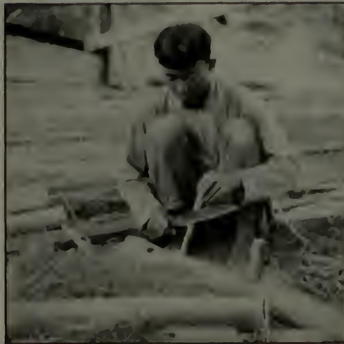
One of the native carpenters making bamboo nails
