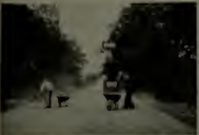
Putting the material on ground for curing
