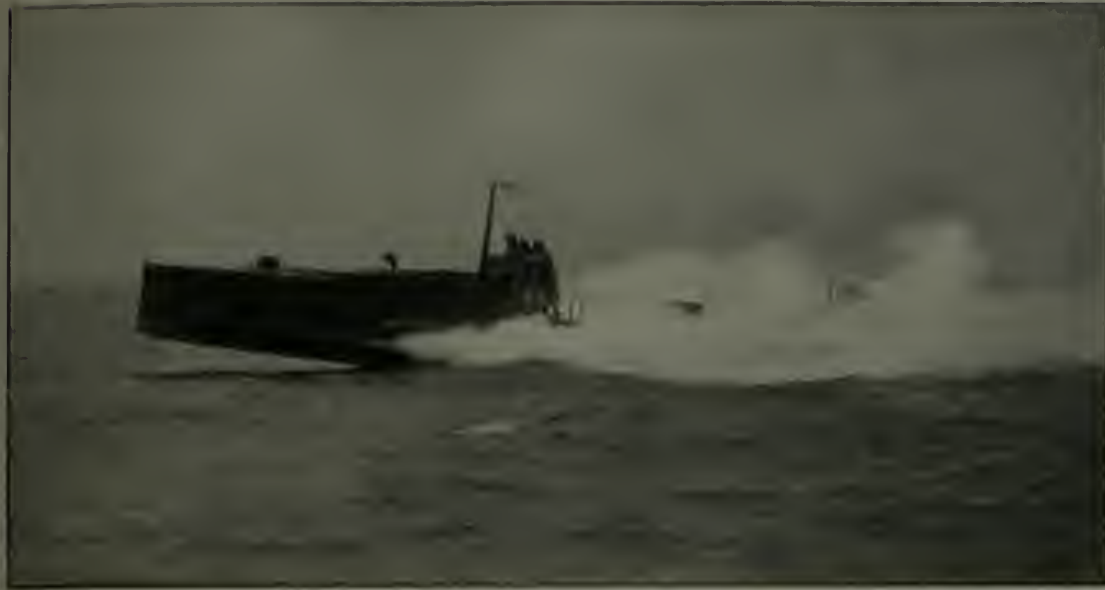
A new motor torpedo boat. She carries an 18-inch tube aft and a rapid-fire gun forward
