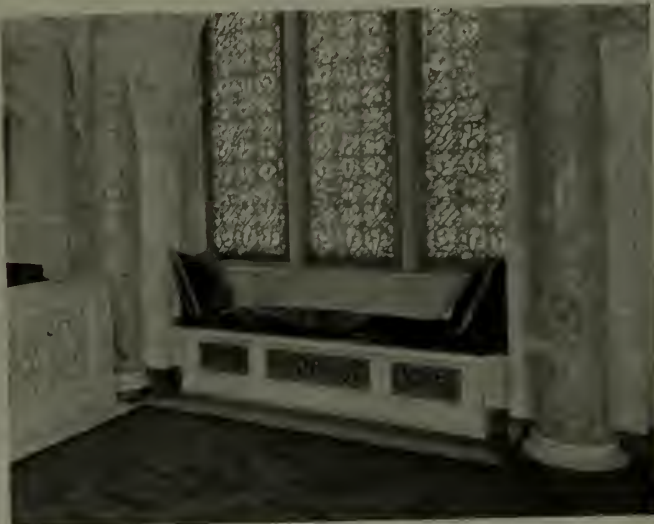
Grille enclosed window radiator in residence of Arthur Curtiss James, New York. Allen & Collens, Architects.
