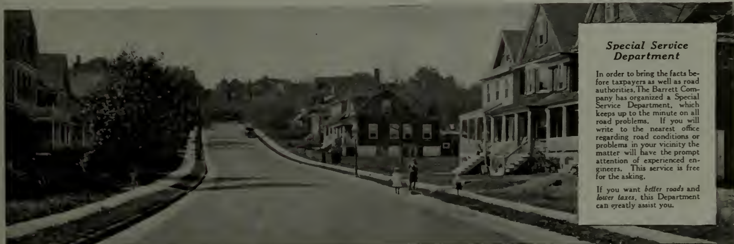
Chauncey Avenue New Rochelle, N. Y. Constructed with "Tarvia-X," 1915. The dustless mudless and automobile-proof surface is very popular with the residents.
