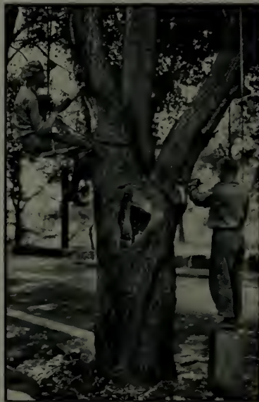
Fig. 2. Same tree with filling removed, showing mass of decayed wood behind the cement
