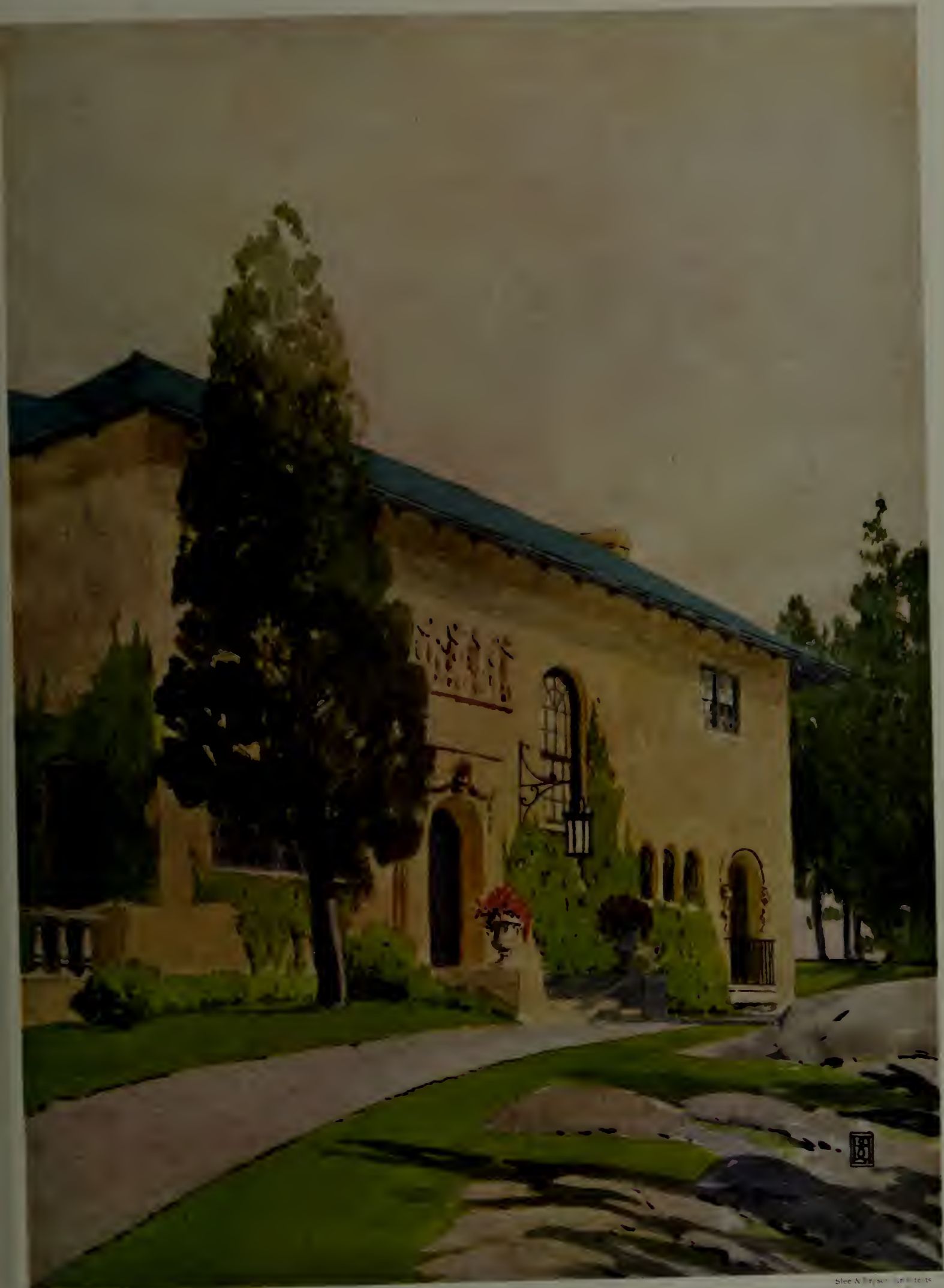
Casa del Ponte, Tokeneke, Conn., with which Mr. Long has taken liberties in the coloring. With the Italian style we associate a freer use of strong colors than are expected in less sunny climates. A typical combination is a wall of salmon pink stucco with a dull blue trim and dark blue tile roof
