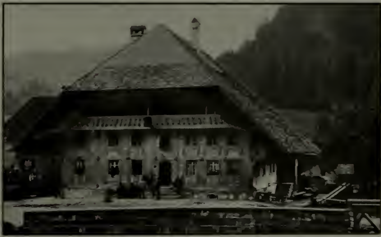
The Bear Inn near Barau. Note arrangement of boards in panels between framing timbers.
