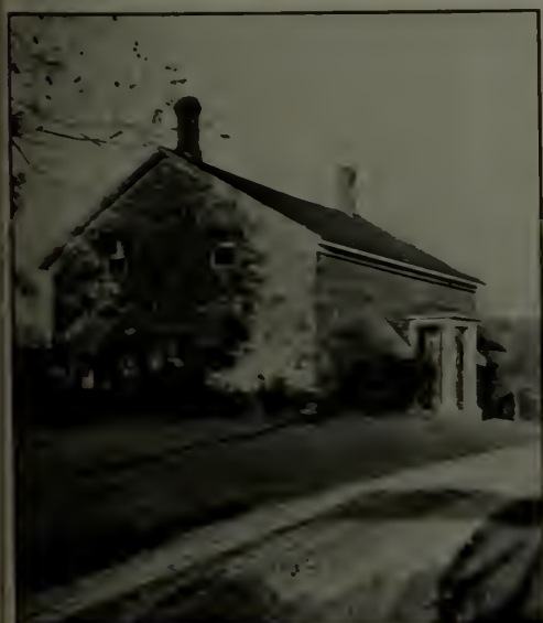
The cobblestones used for building are reddish-brown in color, and they are beautifully rounded and water-worn
