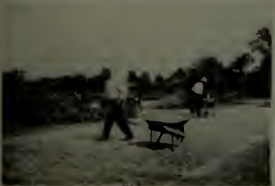
Distributing three-quarter inch stone over the first coat of Tarvia
