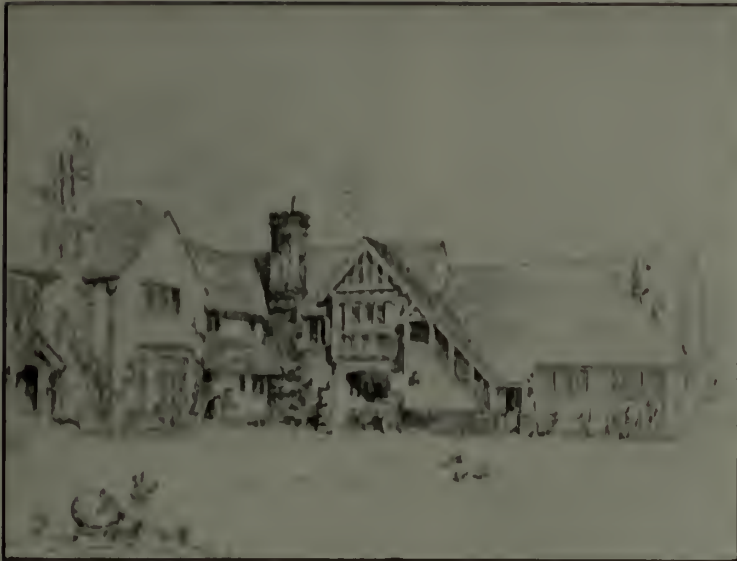
Showing medieval precedent—English type in the house and French in the garage. The gable and outside stairs are reminiscent of old Norman farmhouses. Allen W. Jackson, architect
