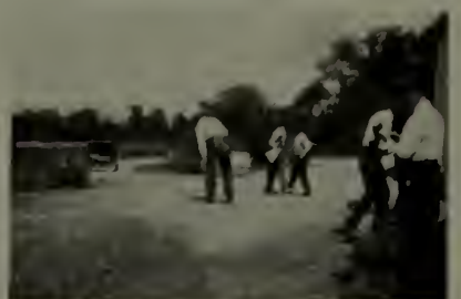
Covering the seal-coat of Tarvia with screenings
