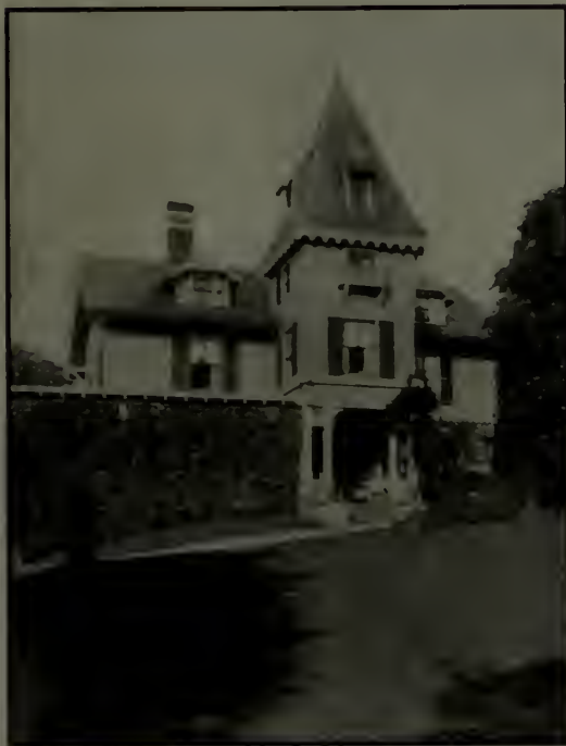
A characteristic Victorian monstrosity, built about 1860 or 1870, belonging to Mr. Charles Hoadley.
