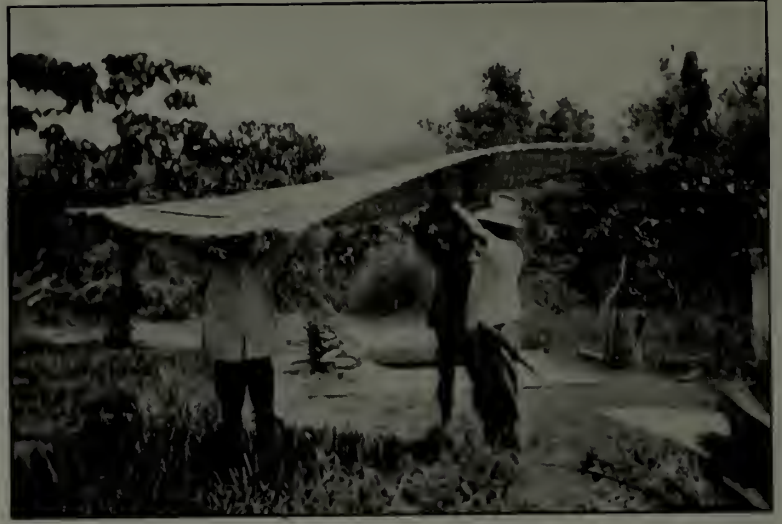
A panel of the wall being lifted into place
