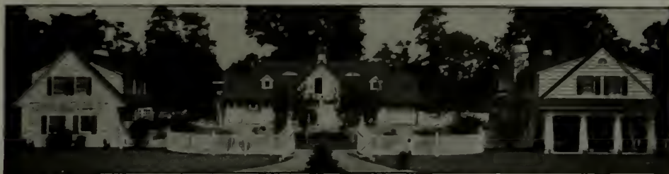
Walls finished with Cabot's Old Virginia White; roofs stained with Cabot's Creosote Stains. Tooker & Marsh, Architects, New York
