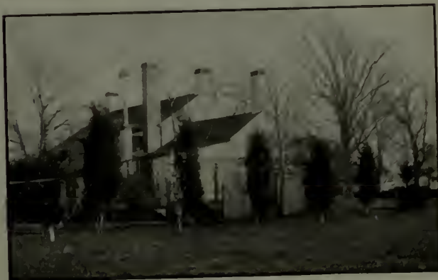
As the Fry house originally appeared from the garden
