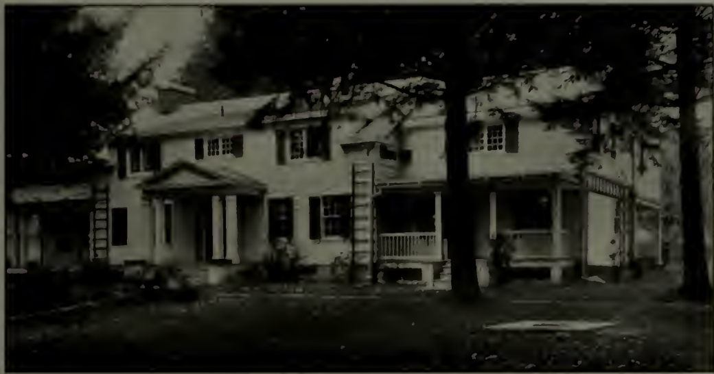
A house at Chappaqua, N. Y., built about 1820, remodelled by Mr. Alfred Busselle. Originally the second story was nothing but an attic, but Mr. Busselle raised the roof to get a full story, built an addition in the rear, removed a narrow porch which ran all the way across the front, and built a new entrance, using for it the original porch columns.
