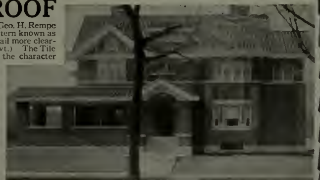
Architects: Postle and Fisher, Chicago, Ill.
