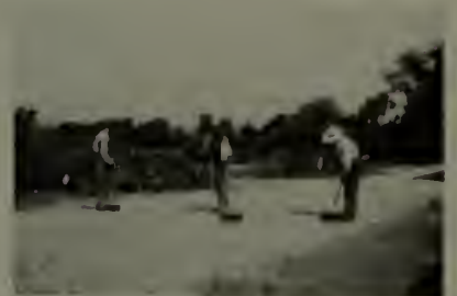
Sweeping off excess of three-quarter inch stone
