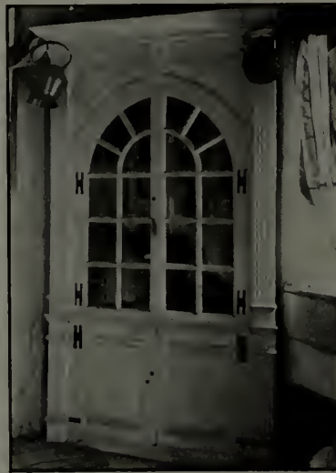
A corner china closet in one of the rooms which owes its beauty to excellent moldings and heavily muntined glass doors
