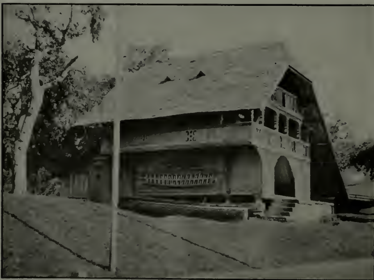
Side and front views of a small house at Barau. Unlike the larger houses pictured above, there are no windows on the first floor, which is given over to storage, the rear lean-to being a stable, while the roof sweeps down to form a shelter for the farm carts
