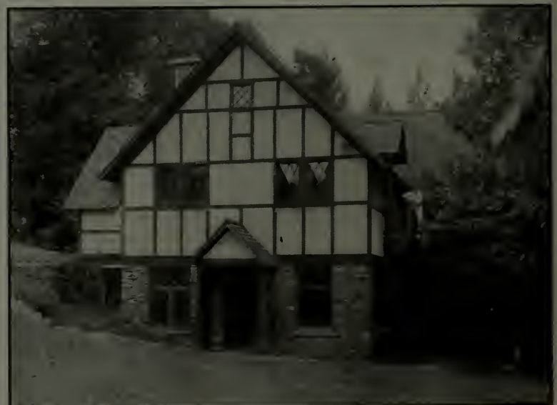
The south side, showing the small latticed porch over the door into the living room
