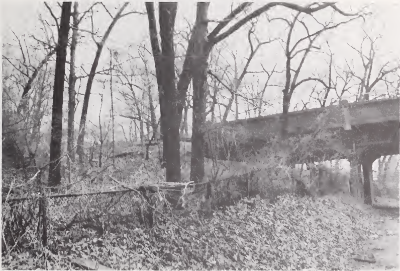
11. Forest Park Drive Overpass
