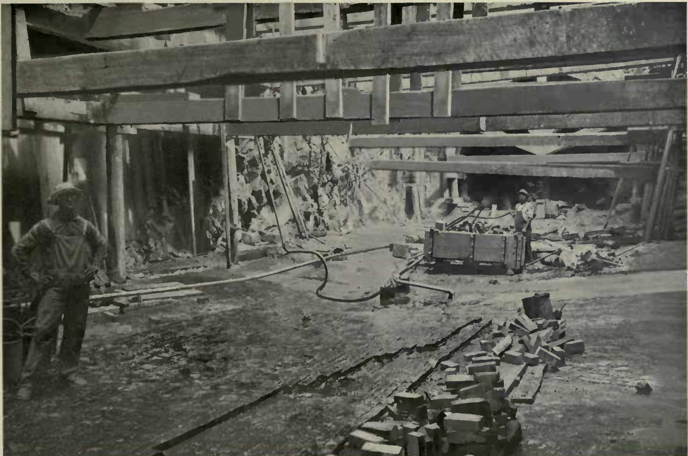
SPECIAL BRICK AND ASPHALT WATERPROOFING
