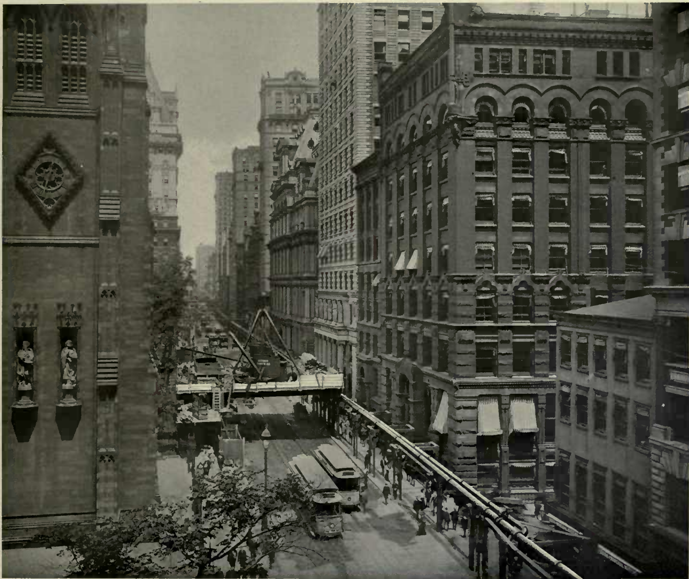
LOOKING UP BROADWAY FROM TRINITY CHURCH — SHOWING WORKING PLATFORM AND GAS MAINS TEMPORARILY SUPPORTED OVERHEAD
