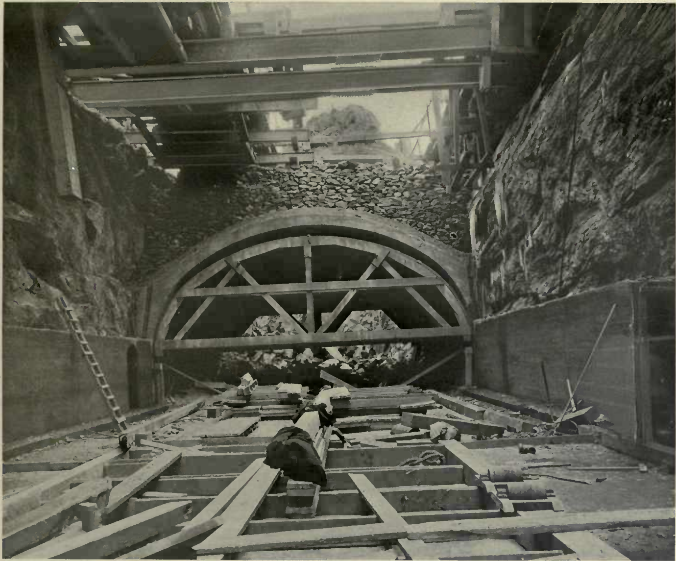
THREE-TRACK CONCRETE ARCH — 117TH STREET AND BROADWAY
