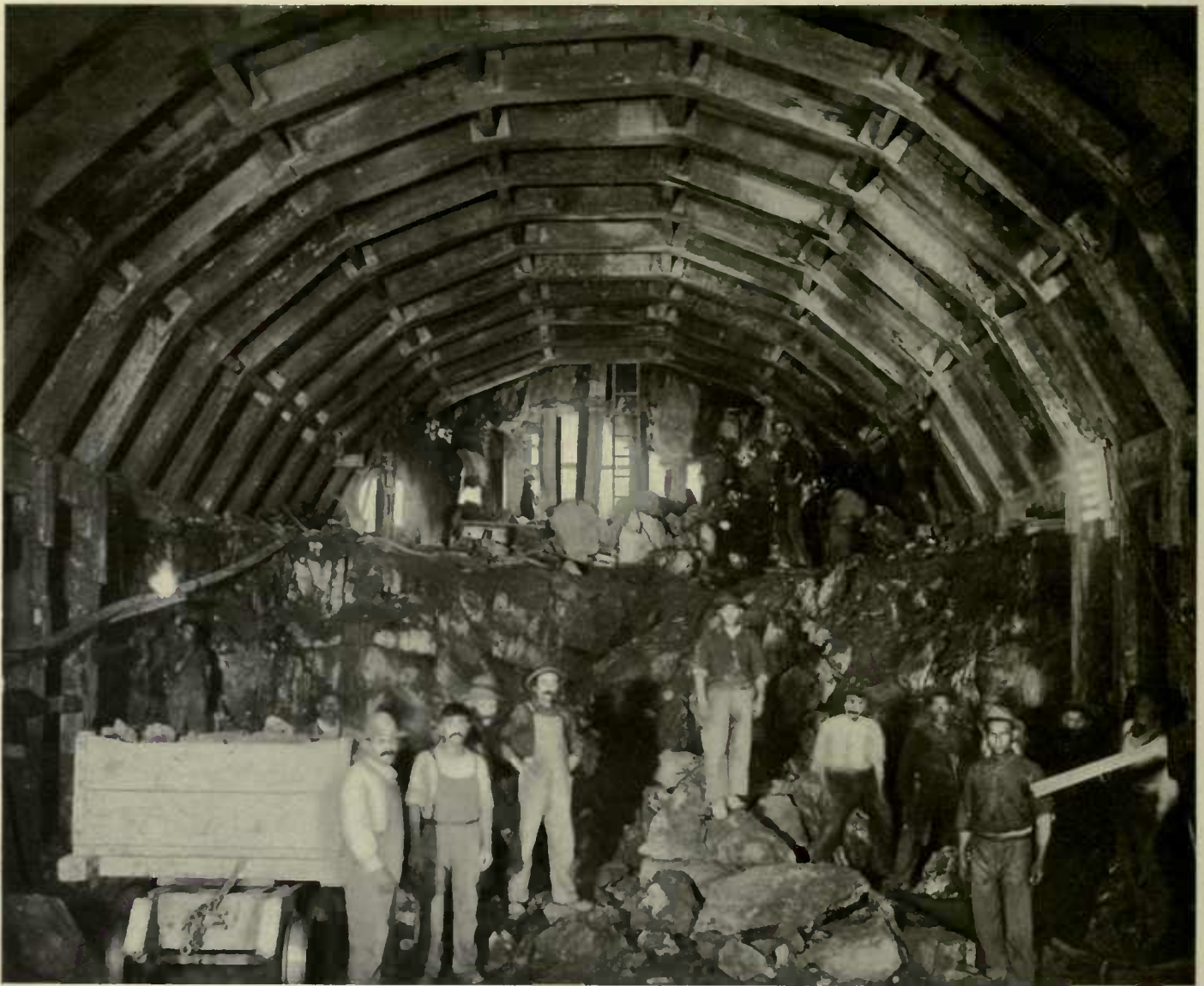
CONSTRUCTION OF FORT GEORGE TUNNEL
