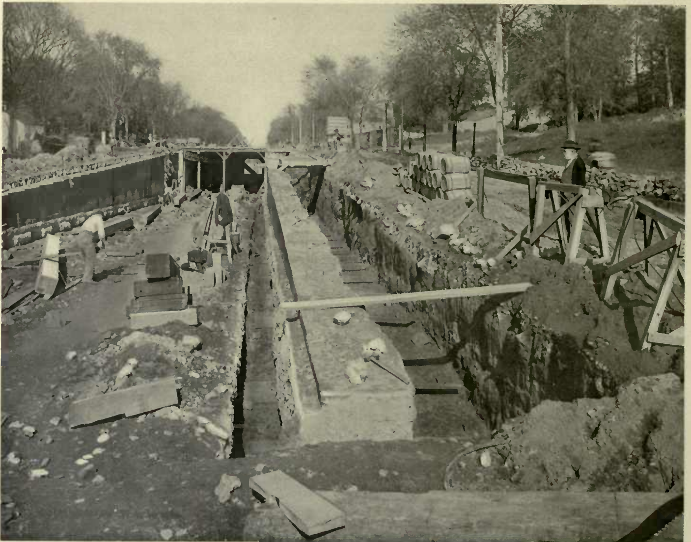
MOVING BRICK AND CONCRETE RETAINING WALL TO MAKE ROOM FOR THIRD TRACK—BROADWAY AND 134TH STREET
