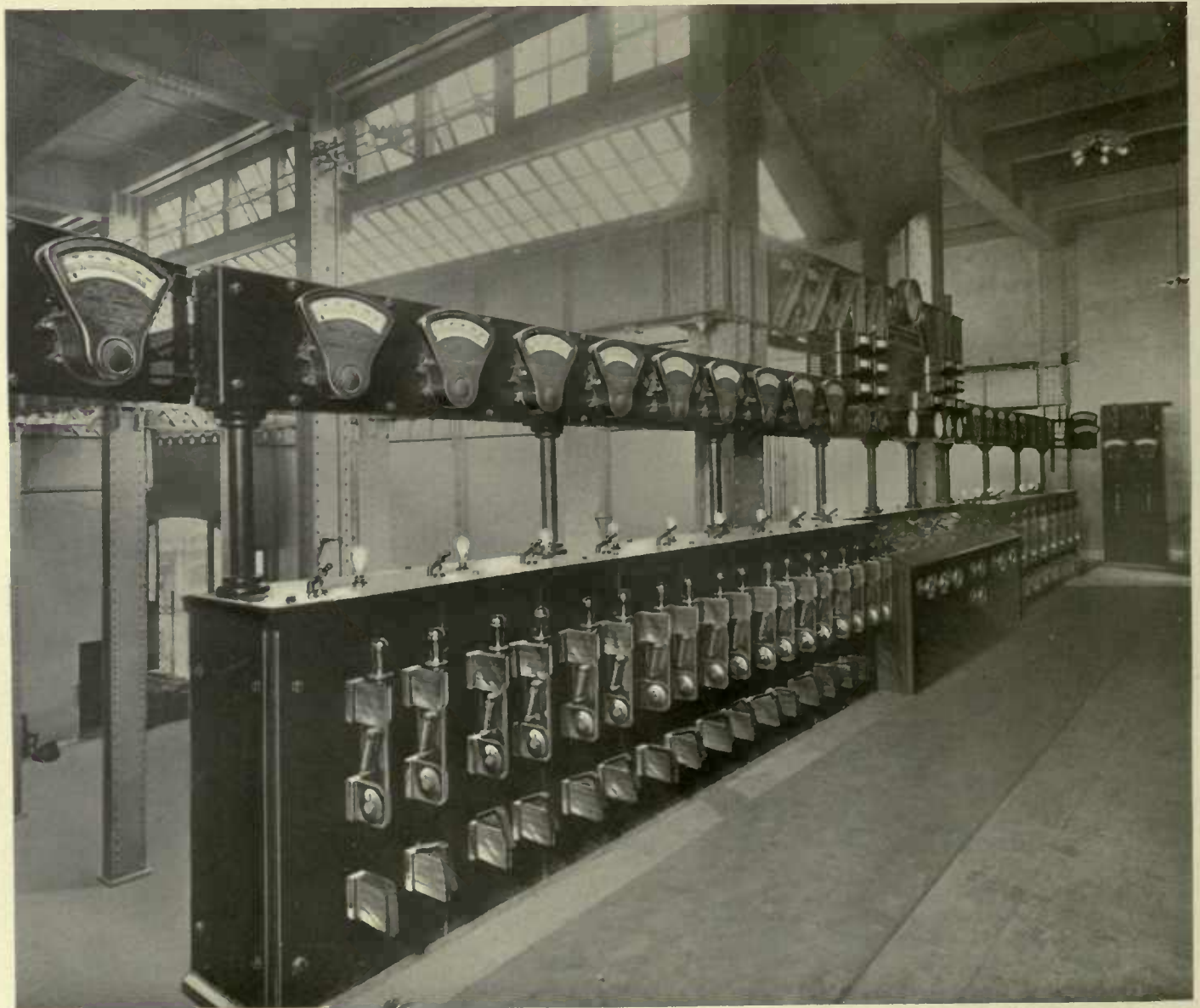
OPERATING BOARD—SUB-STATION NO. 11
