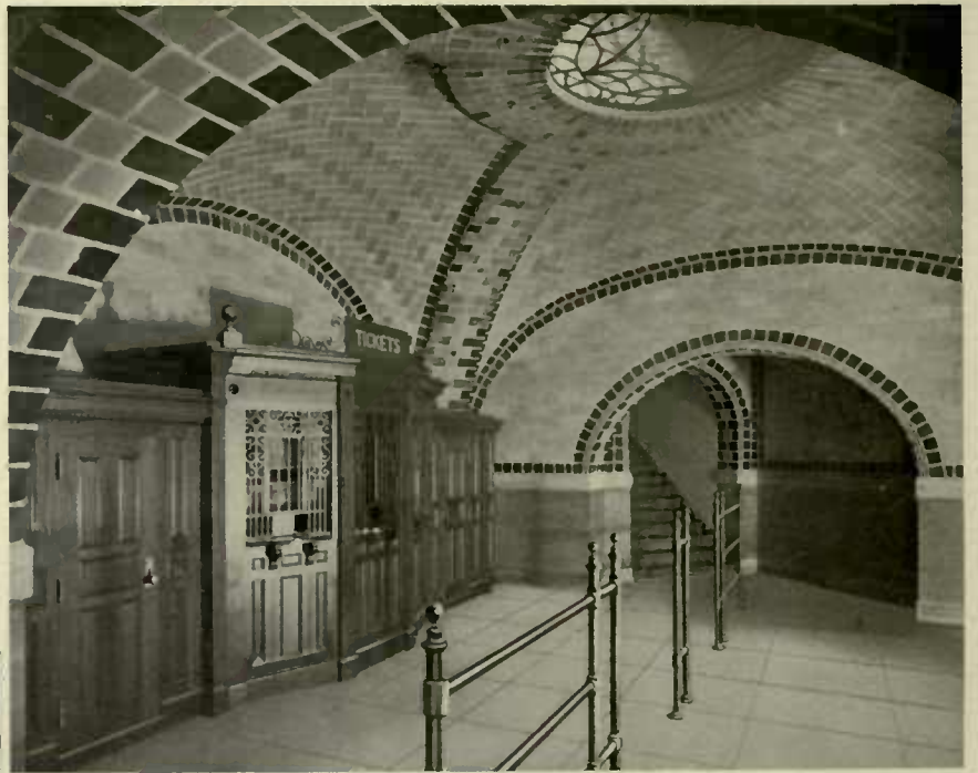
CITY HALL STATION
