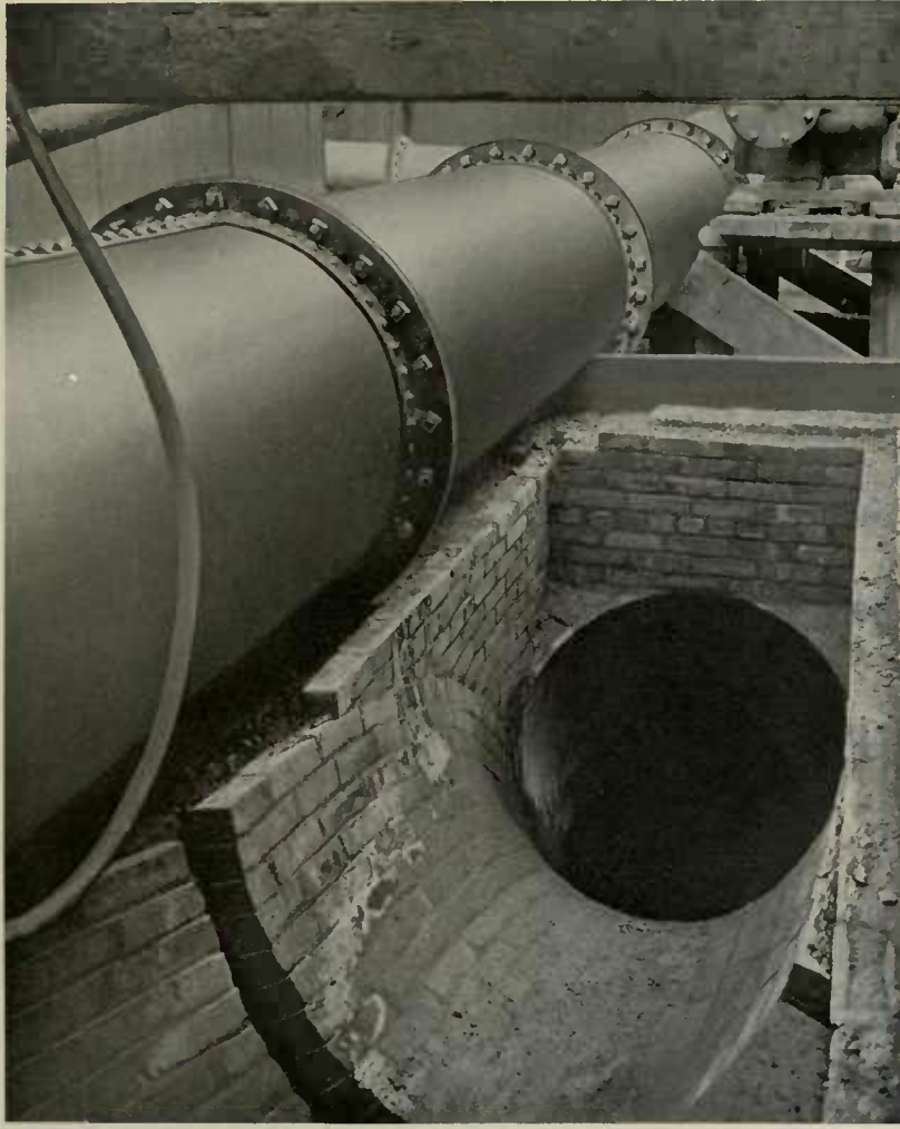
SEWER SIPHON AT 149TH STREET AND RAILROAD AVENUE
