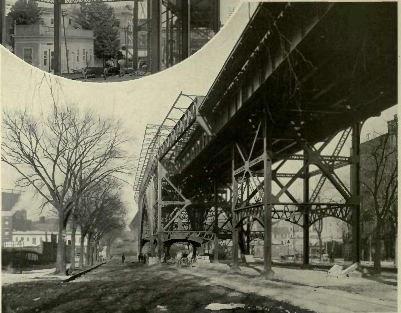
MANHATTAN VALLEY VIADUCT, LOOKING NORTH
