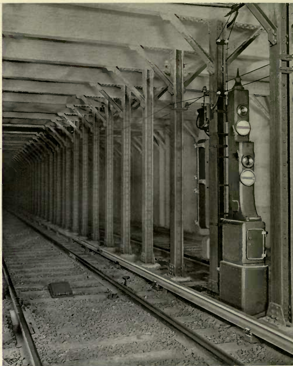
FRONT VIEW OF BLOCK SIGNAL POST, SHOWING LIGHTS, INDICATORS AND TRACK STOP
