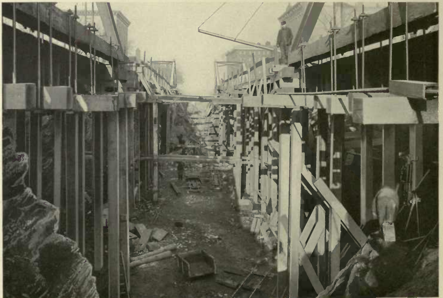
SURFACE RAILWAY TRACKS SUPPORTED OVER EXCAVATION ON UPPER BROADWAY
