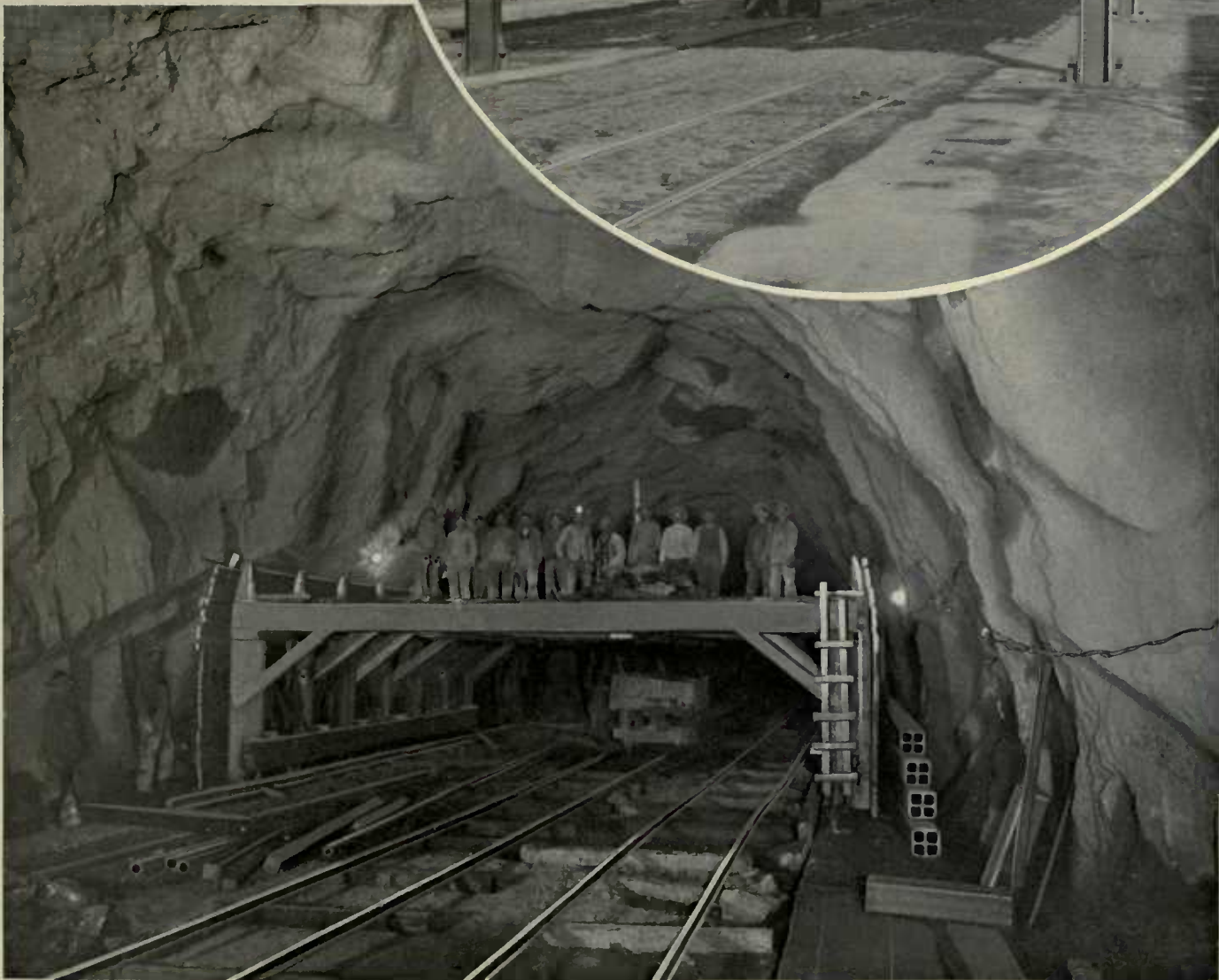
TRAVELER FOR ERECTING FORMS, CENTRAL PARK TUNNEL — (IN THIS TUNNEL DUCTS ARE BUILT IN THE SIDEWALLS)
