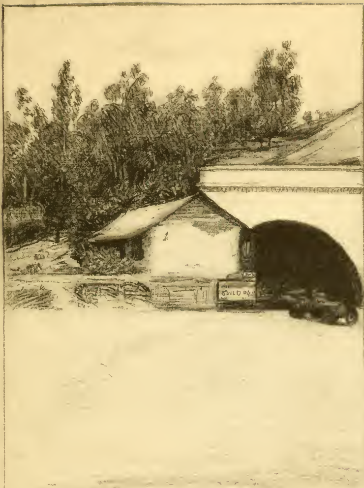
"North End Boatway Tunnel"
