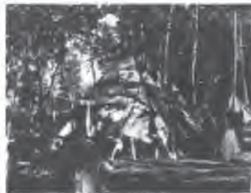
No. 9 Salix (summer light) - these are covered over with the long strips of birch bark (striated) - over a skeleton of staves.
