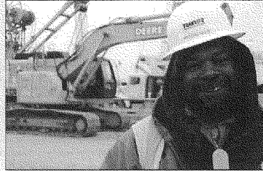
Antoine Blair (above), a construction worker from Washington, D.C., was unemployed when he was hired to help DC Water improve its pollution control systems. "It's creating a lot of jobs," he said.
