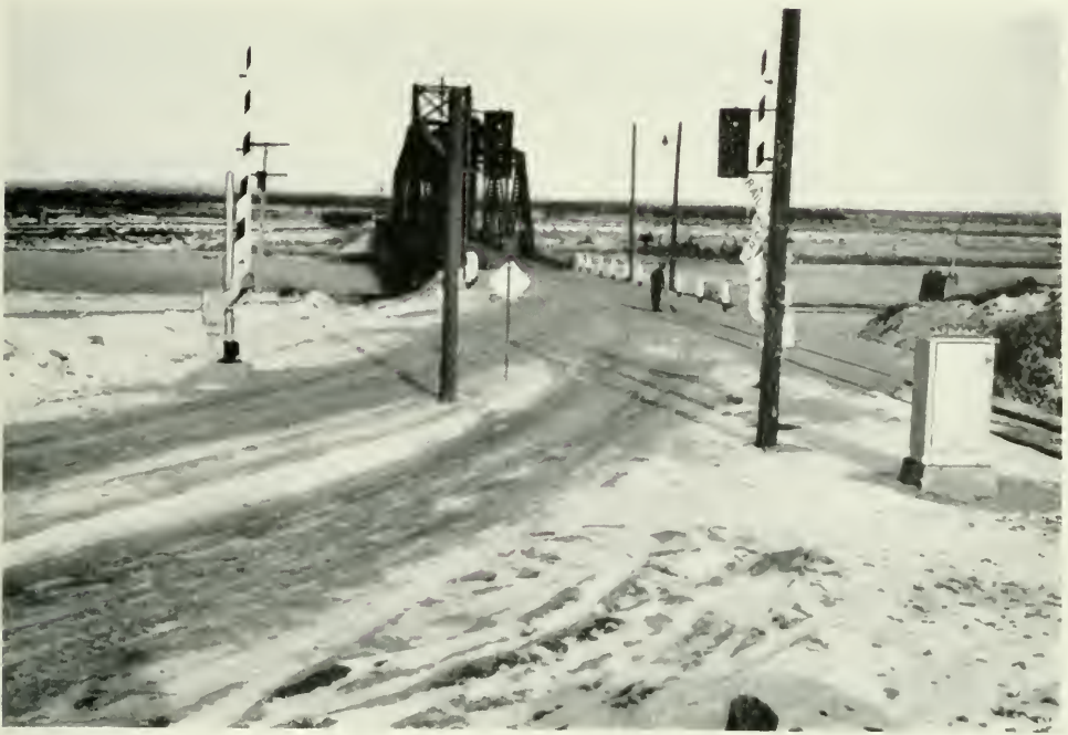
Approach to bridge at Little Current, showing traffic signals to control both train and motor vehicle traffic.
