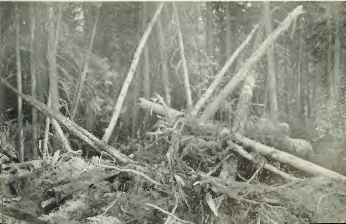
Excessive waste from bulldozing a road before cutting the right-of-way. (Pulpwood-exporting company operation.)
