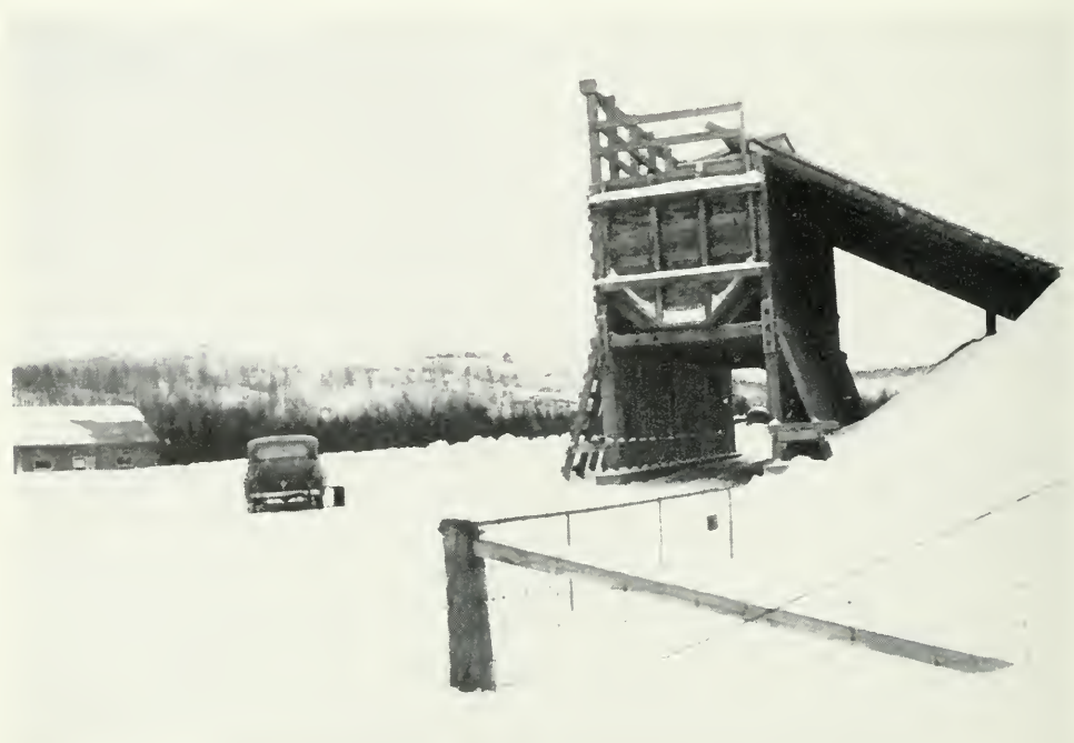
Sand loading bin located at junction of No. 11 Highway and Airport Road near North Bay.
