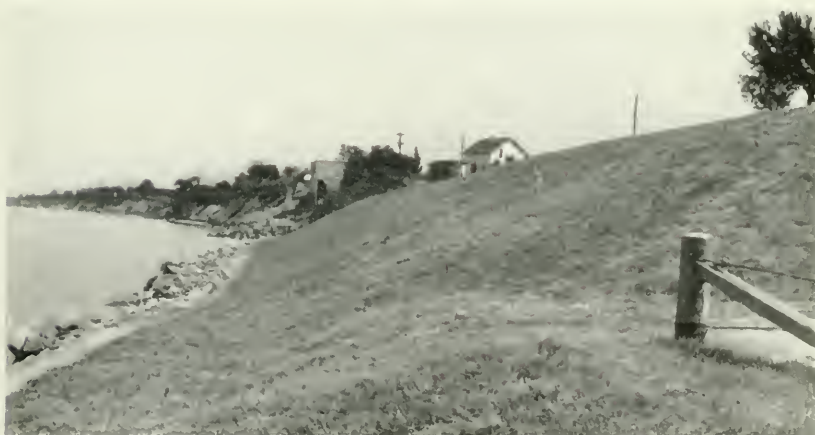
Finished graded and sodded shoreline.
