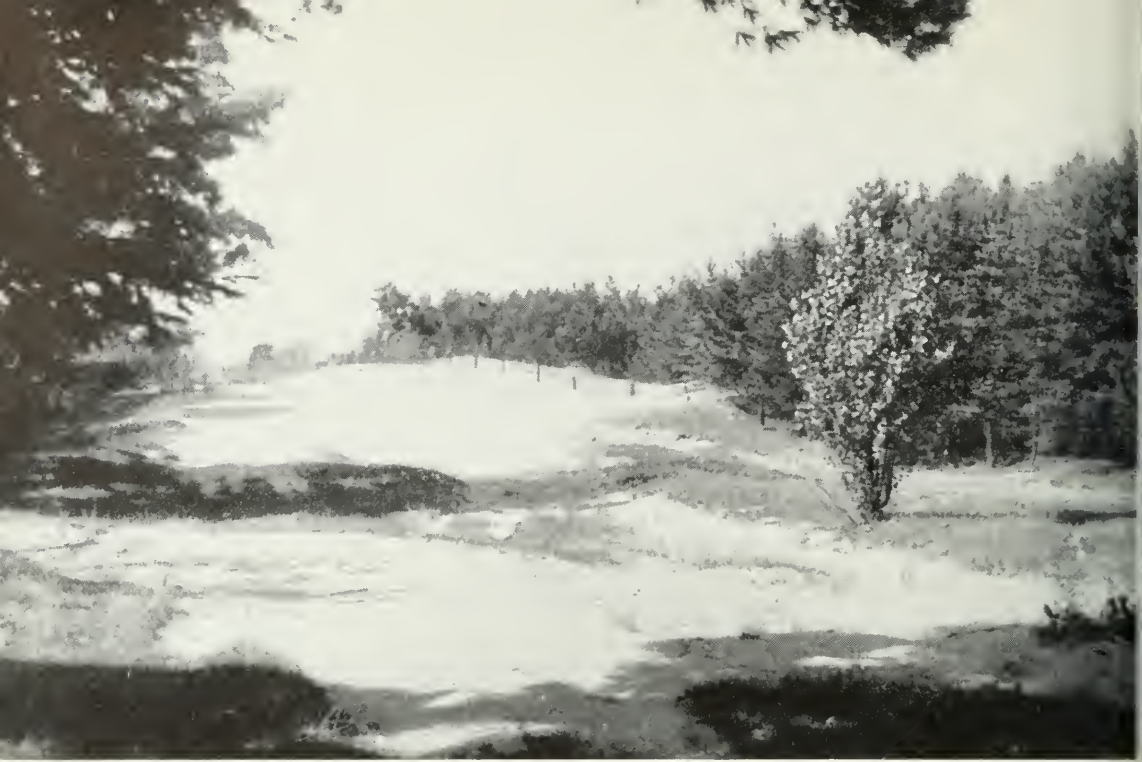
Blow-sand has made this road unfit for use. Note the plantation on the right which is correcting this condition. Ontario County.
