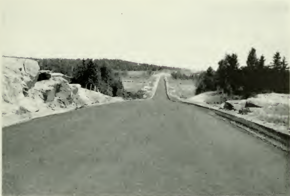
Mulch surface on new Creighton Mine Road.
