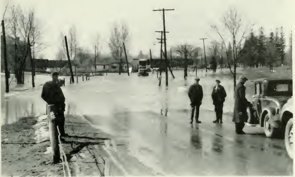
Spring flood conditions on Highway No. 2 at Pickering.
