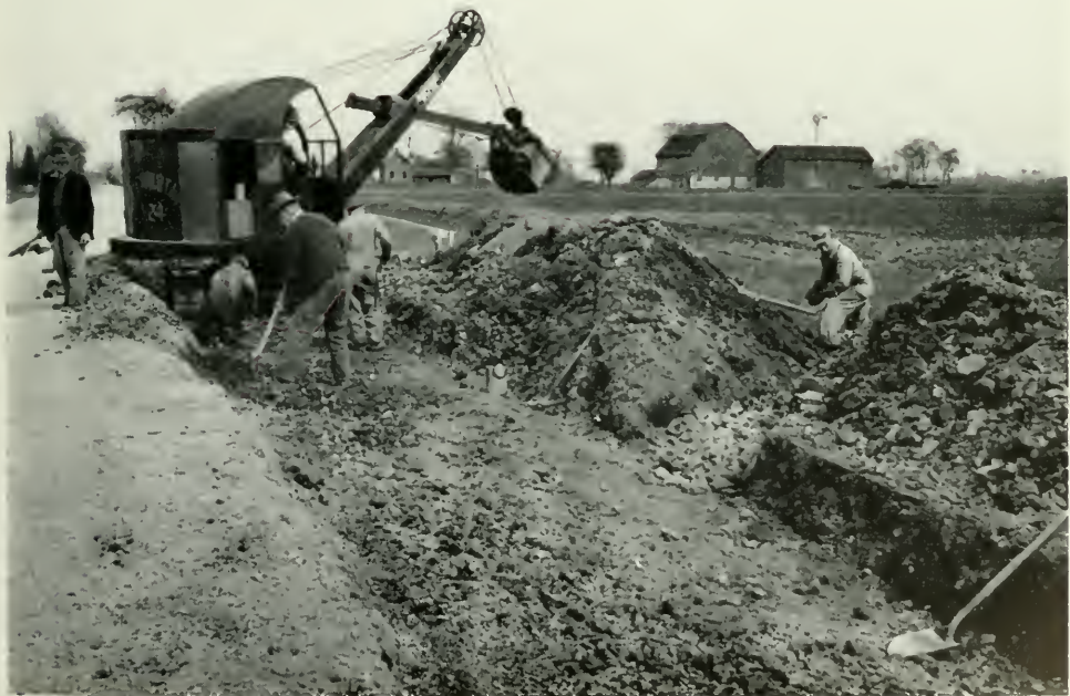
Excavating disintegrated roadbed on Highway No. 3 between Jarvis and Simcoe.
