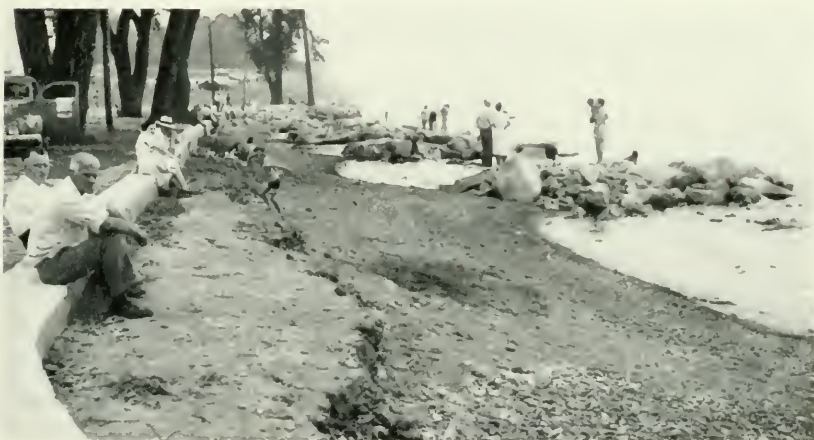
Rock groins built out from shore to build up sand beach.
