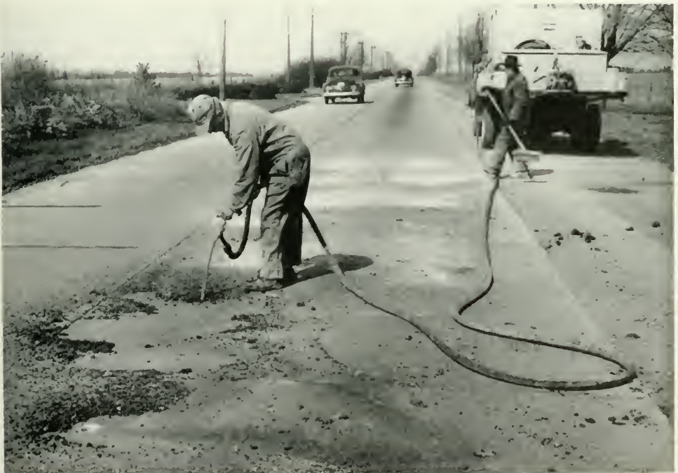
Asphalt jacking operations.
