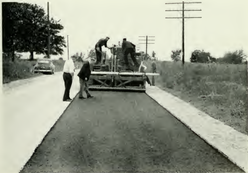
Laying bituminous carpet coat.
