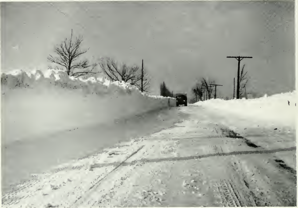
A winter highway widened by rotary plow.
