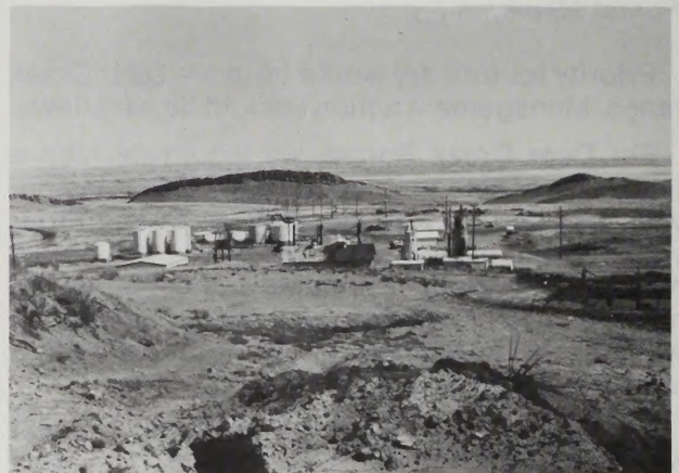
Tank battery, oil and gas processing facility
