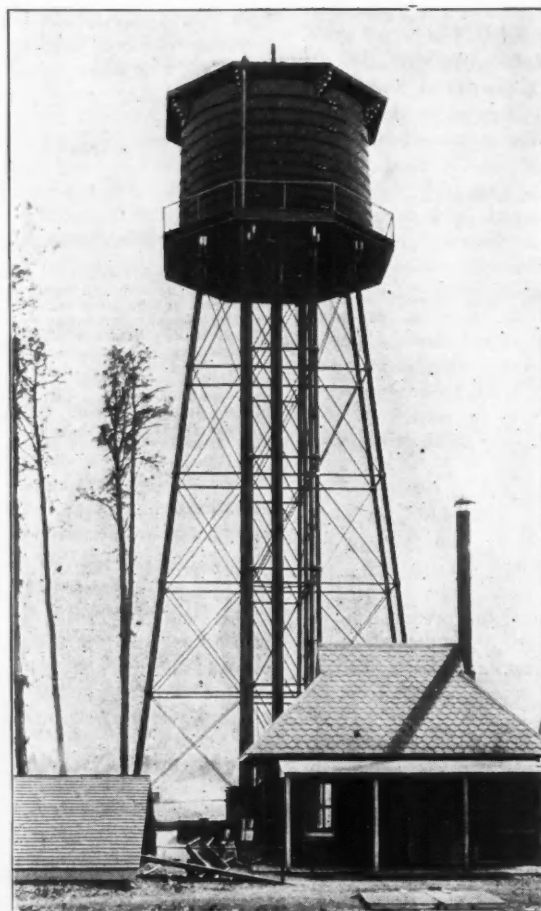
TANK OF 50,000 GALS. CAPACITY AT ALLENHURST, N. J.
