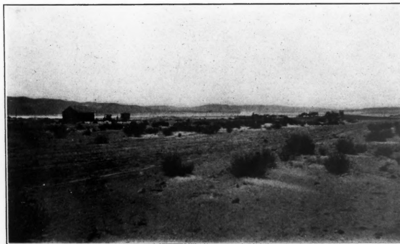
SAND WELLS STATION ON ROAD
