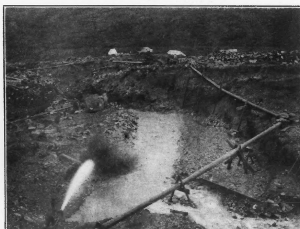
FIG. 7. HYDRAULICKING FROZEN GRAVEL
