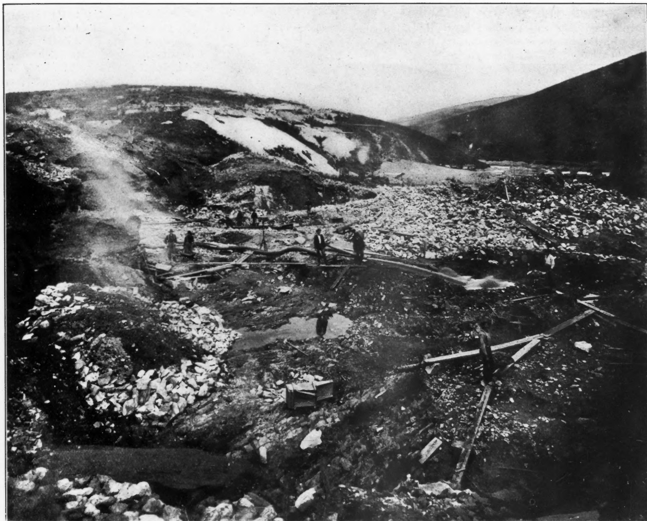
FIG. 11. HYDRAULICKING WITH PUMPED WATER
