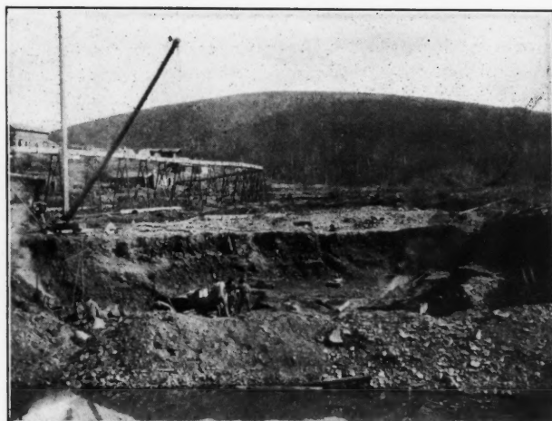
FIG. 6. OPEN CUT WITH HOISTING DERRICK
