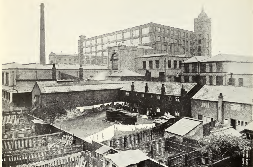
PLANT AT LEIGH, NEAR MANCHESTER, SHOWING MAGNIFICENT MILL AND WRETCHED TENEMENTS
