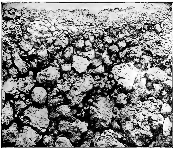
Fig. 25. Photograph showing a section of soil not fined nor compacted below.
